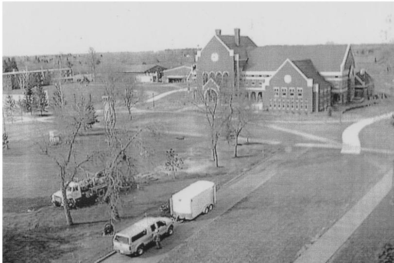
Figure 4 - Drilling of boreholes
