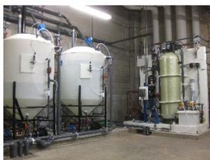
**Grey Water System** In 2011, The Williams Village North Residence Hall was constructed and includes a greywater system estimated to save 700,000 gallons of water a year. The non-potable water system harvests used water from showers and sinks, treats it, then reuses it for flushing and cooling tower make-up.
