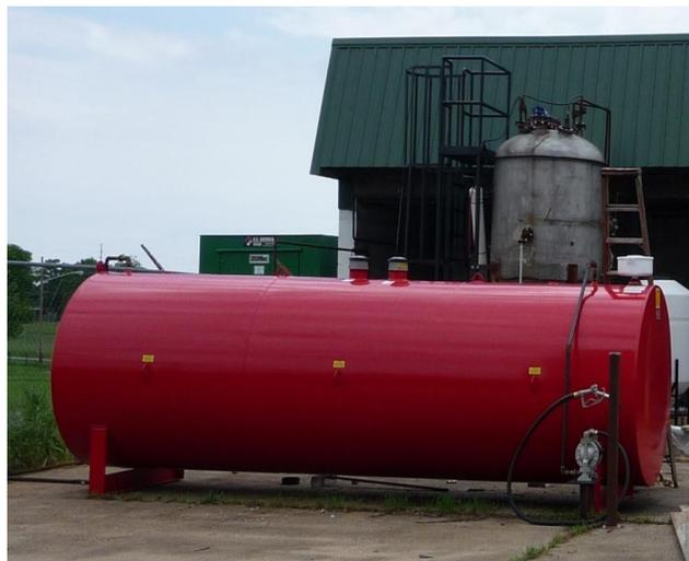
Figure 4: Final Biodiesel Storage Tank
