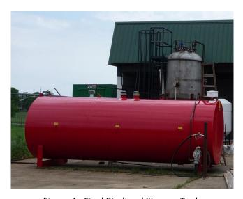
Figure 4: Final Biodiesel Storage Tank
