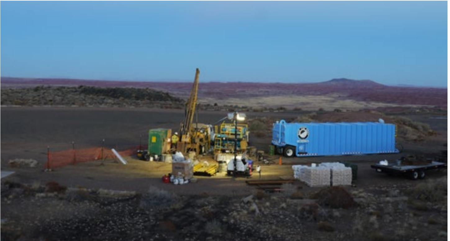
Moonset at CPCP drilling site
