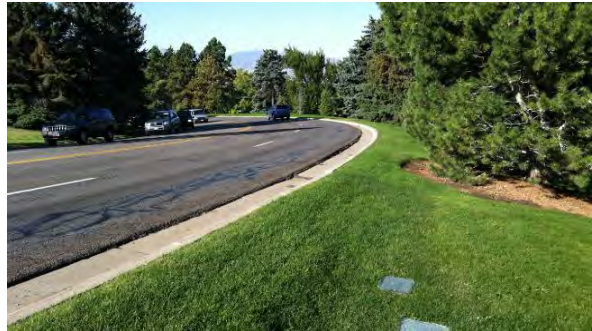
Looking west along North Campus Drive where the road turns to the south; grade and utilities may pose challenges
