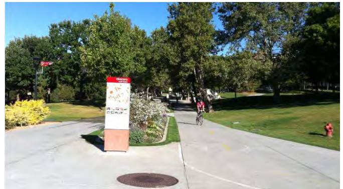
The existing split configuration of the bike and pedestrian portions of the corridor
