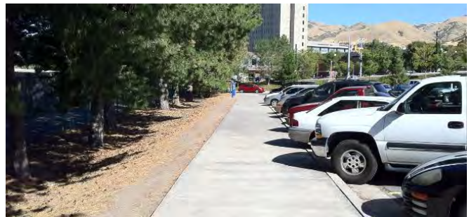
Wheel stops should be added to the parking lot
