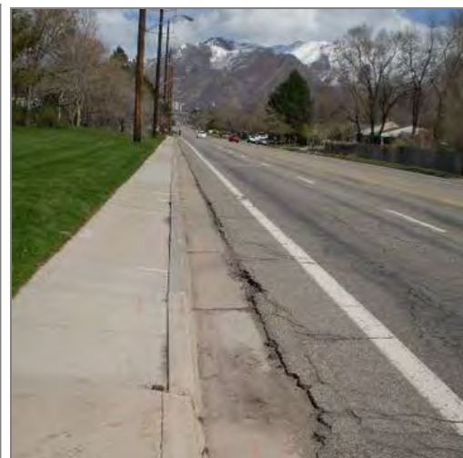
(Left) The Foothill Drive shared-use path crosses six lanes of dense traffic on Wakara Way to reach a refuge area; finding a gap is difficult during peak periods (Right) the Sunnyside Avenue bike lanes are narrower than AASHTO minimum widths and have a deteriorating gutter seam
