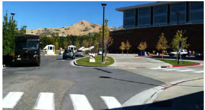
The curb ramp should be widened in front of the library
