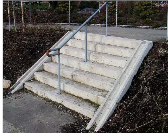
Bike “channels” or “troughs” allow bicyclists to walk their bicycles up/down staircases as opposed to carrying them.
