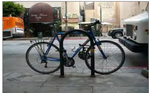
Inverted U bicycle racks provide enhanced stability and security by supporting the bicycle frame at two points
