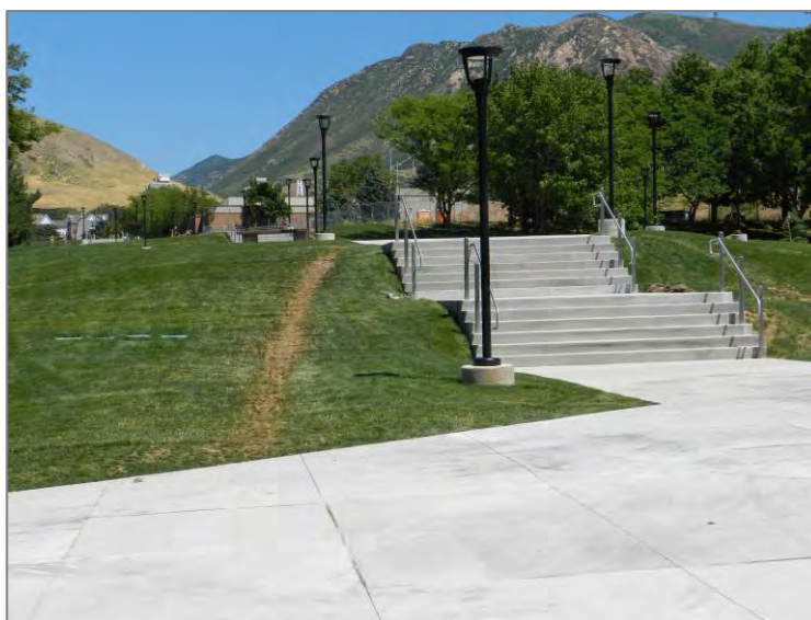
Grass is worn by bicyclists bypassing the stairs just weeks after installation.
