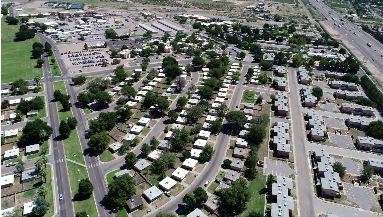
Figure 4 | South Residential Housing Area
