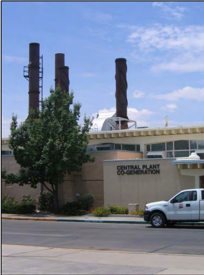
Figure 10. NMSU Central Plant.
