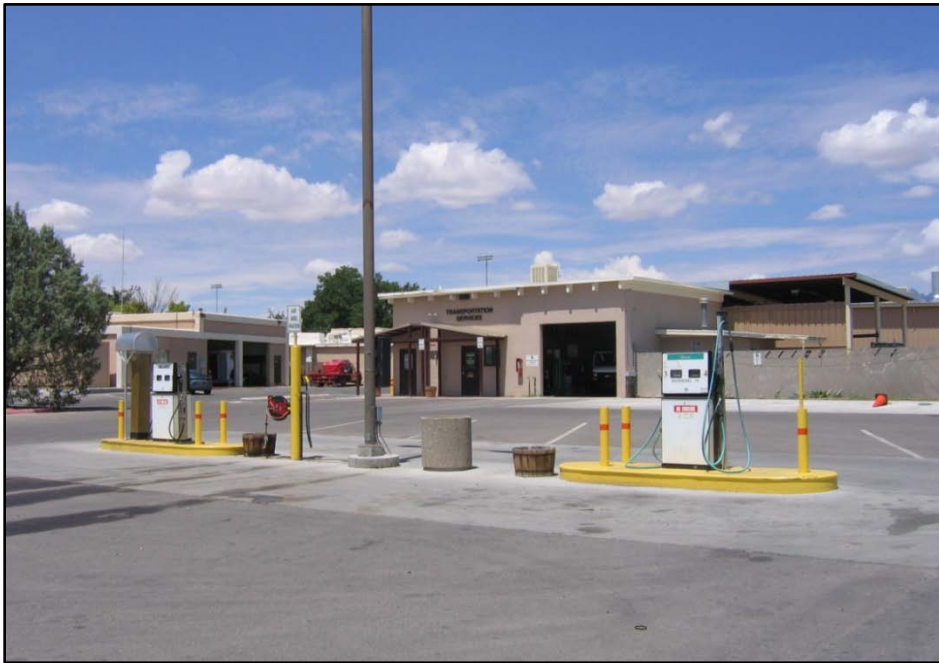
Figure 9. Fleet Maintenance Facility.
