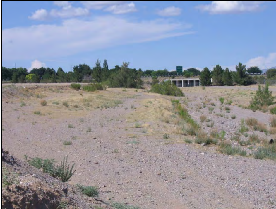
Figure 3. Tortugas Arroyo, Looking Upstream from Wells Street.
