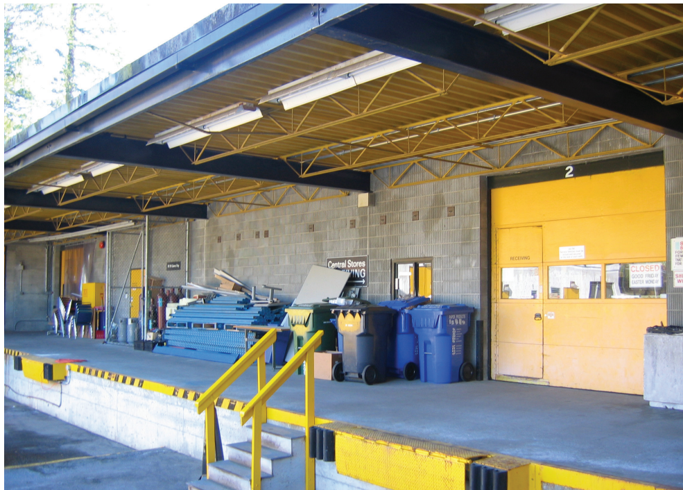
figure C-3: Central Stores Loading Bay
