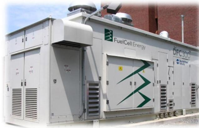
*250-kW Molten Carbonate Fuel Cell - SUNY ESF*
