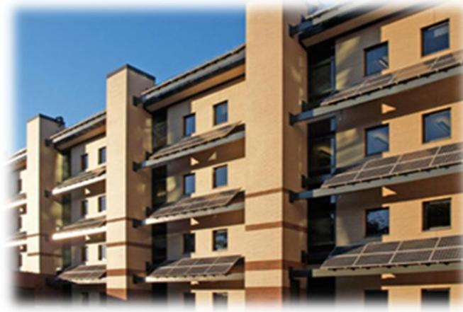
*25-kW Solar PV Array, Baker Lab - SUNY ESF*
