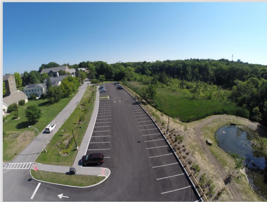
Olin Parking Lot, Bard’s 2015 permeable asphalt parking lot designated for Commuters only, with reconstructed wetland and drainage system. ( LRC Associates, 2015 )
