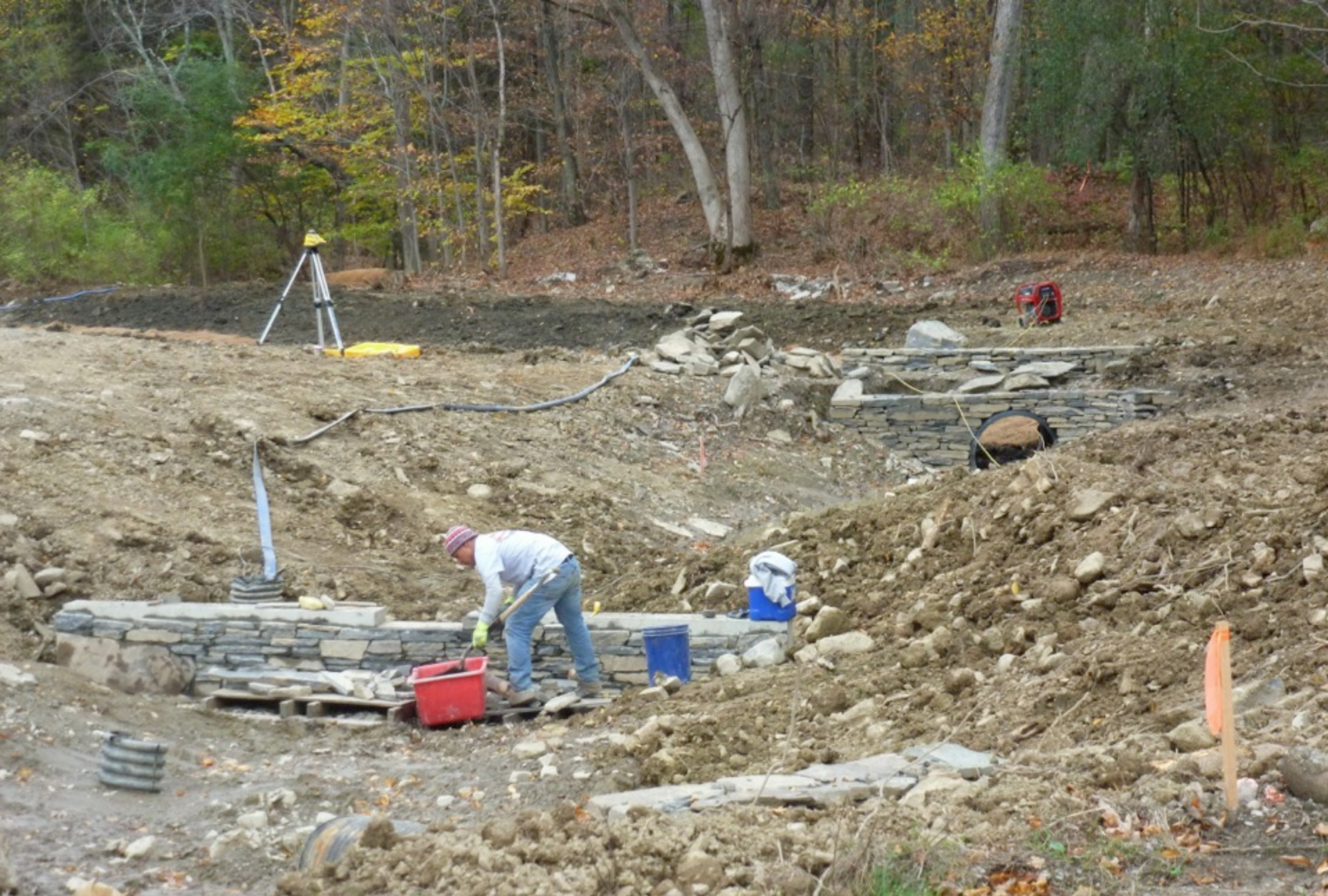
CONSTRUCTION OF THE WEIR WALL AND WETLAND CROSSING
