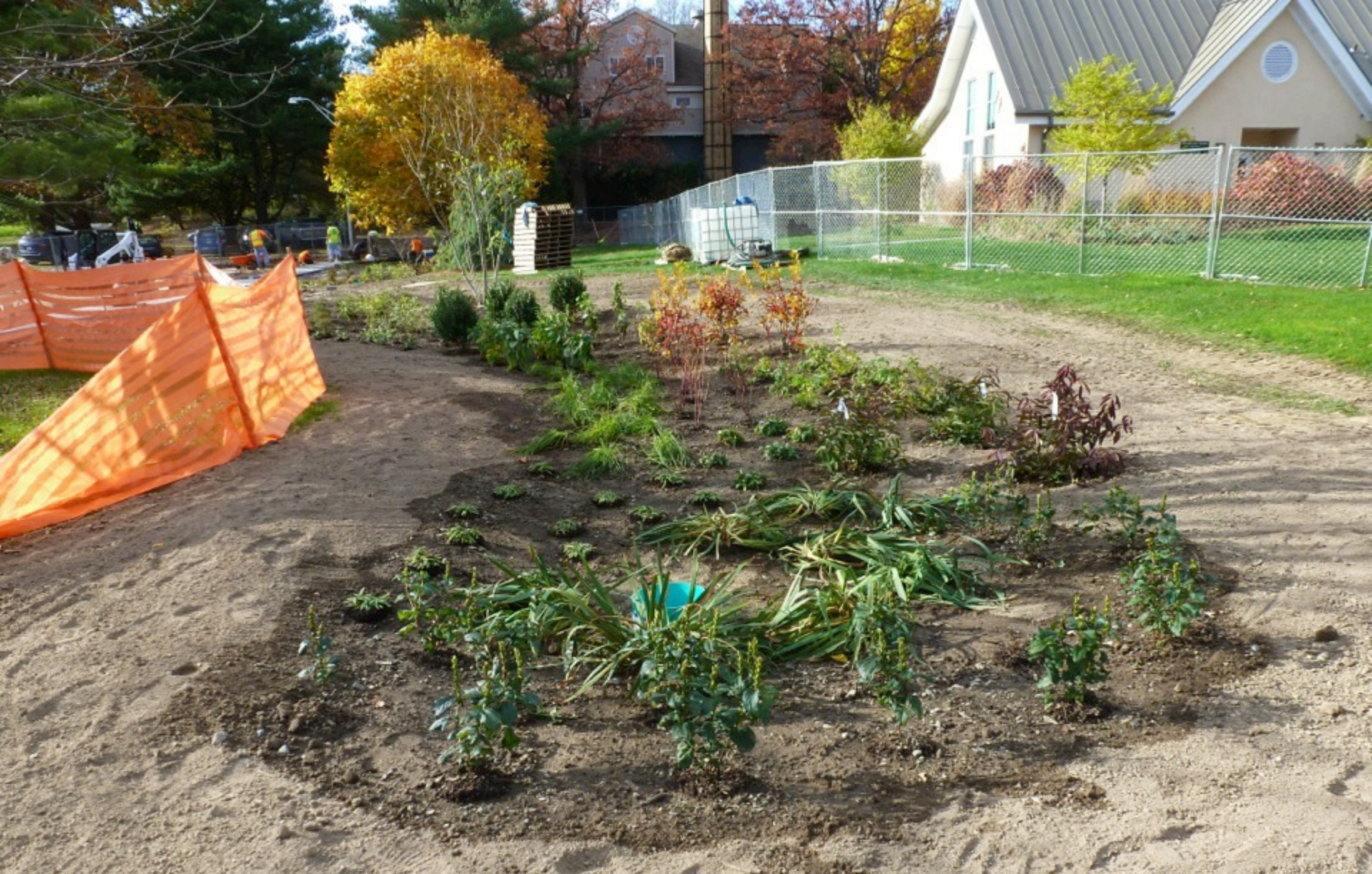
ONE OF THE BIORETENTION AREAS JUST AFTER INSTALLATION
