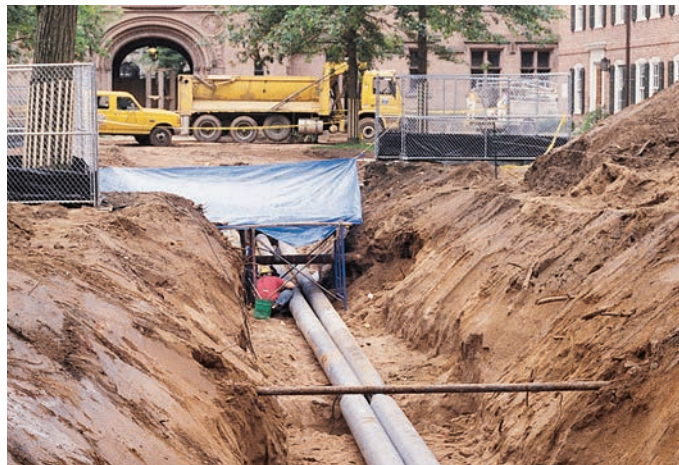
Utilities: Installation of underground conduit on Core Campus
