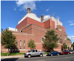
Cogeneration at Central Power Plant
