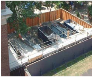
Construction and demolition waste properly sorted for recycling
