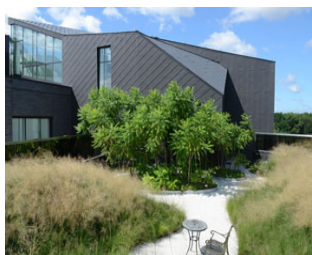
Green roof at Yale Health Center reduces stormwater runoff
