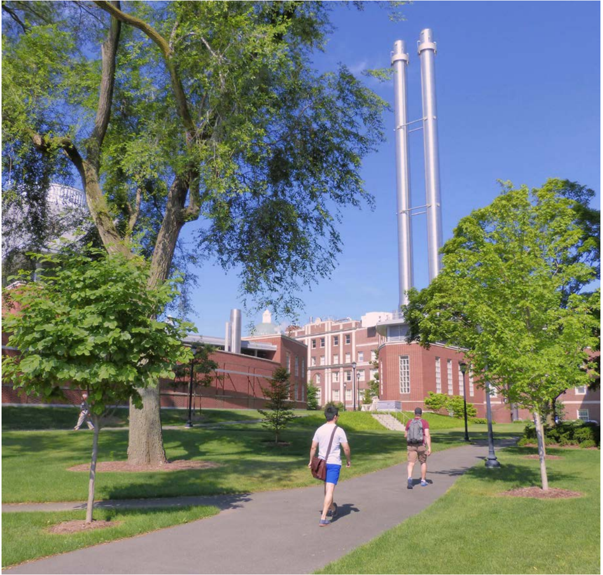
The cogeneration facility at Sterling Power Plant is highly efficient saving up to 18,000 metric tons of carbon equivalent per year.
