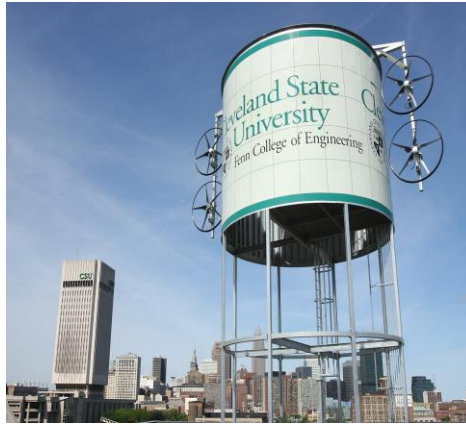
Figure 1- Functional CSU's Wind Tower Installed at Campus
