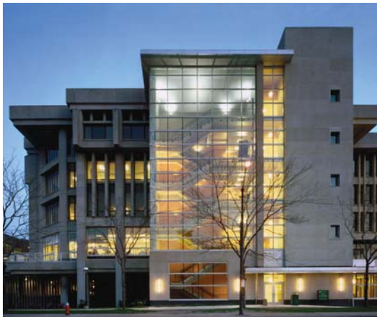
Figure 87: Main Classroom, new entry tower
