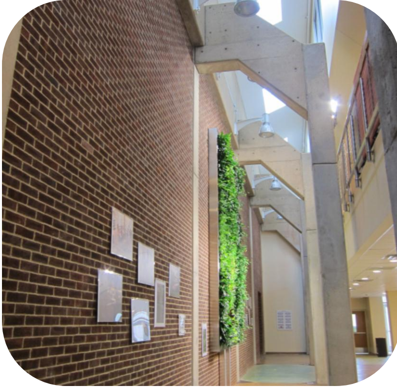
Figure 4 Reused exterior wall now interior; skylights above
