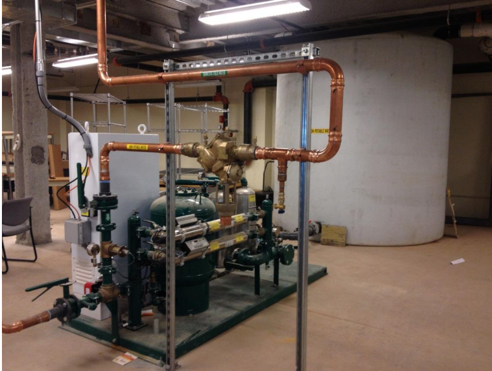
Figure 3 Rainwater harvesting system
