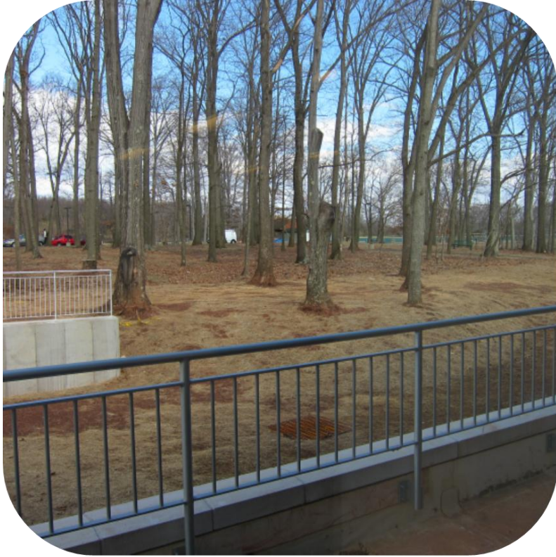
Figure 5 Showing tight construction site footprint
