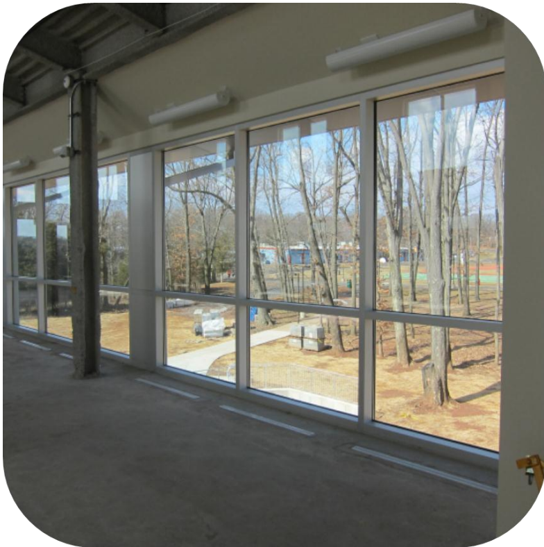
Figure 6 View from unfinished third floor window wall
