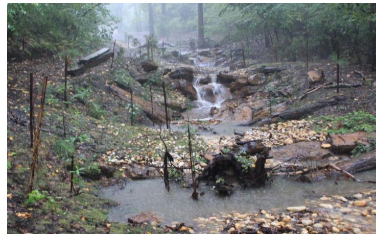
Example of a Completed Outfall and Stream Restoration Project – Photo Credit Biohabitats, Inc.
