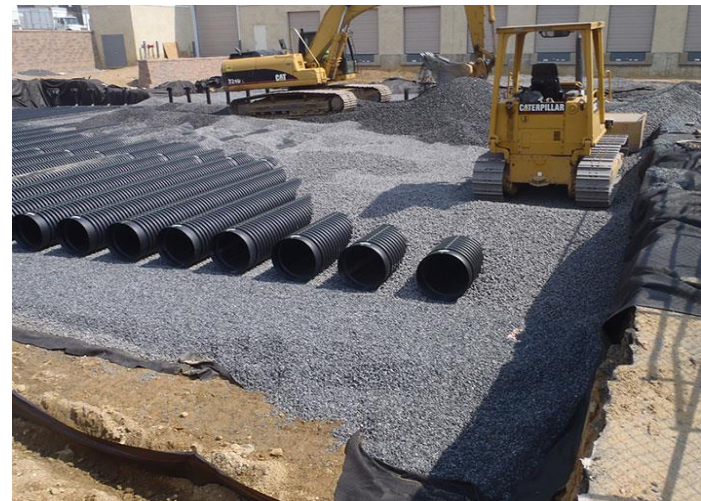
Subsurface Infiltration Bed
