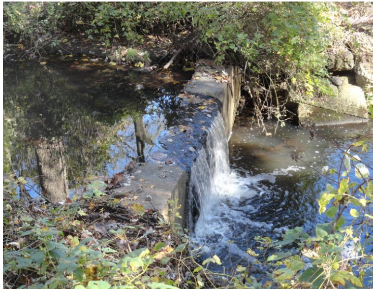
Concrete Weir in Stream Near Nature Trail
