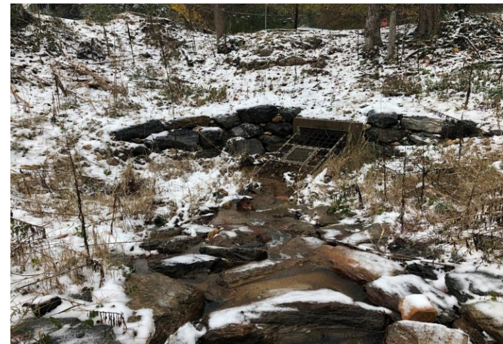
Wedge Shaped Debris Rack Installed Upstream of a Culvert Entrance
