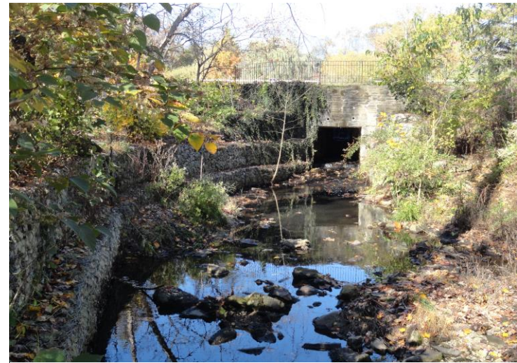
College Lane Culvert and Streambank Protection
