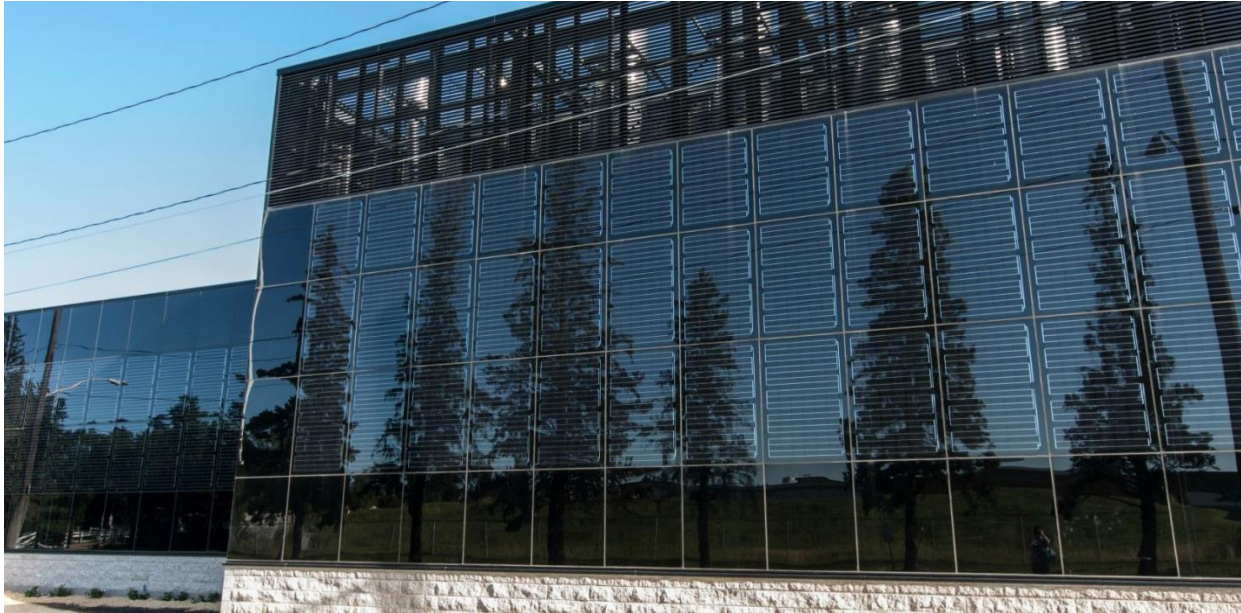
Figure 3. Building-integrated solar PV at the Medical Isotope and Cyclotron Facility.
