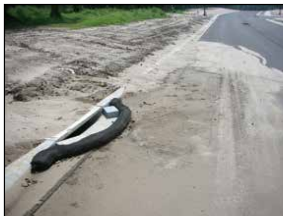
Drain Inlet Protection
