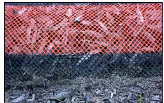
Close Up of Sediment Control
