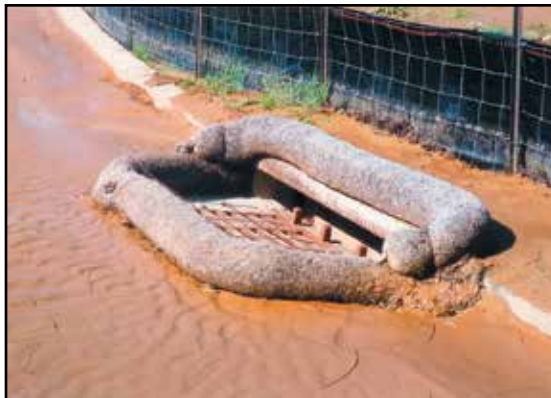
Curb Inlet Protection – Fine Silts Filtration
