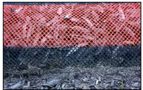
Close Up of Sediment Control
