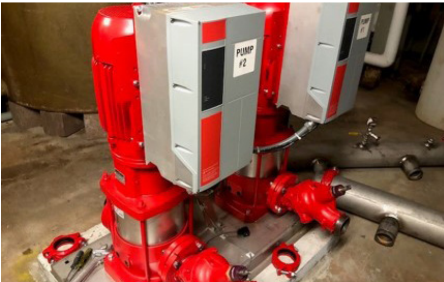
Photo 4. High efficiency pumps being installed
