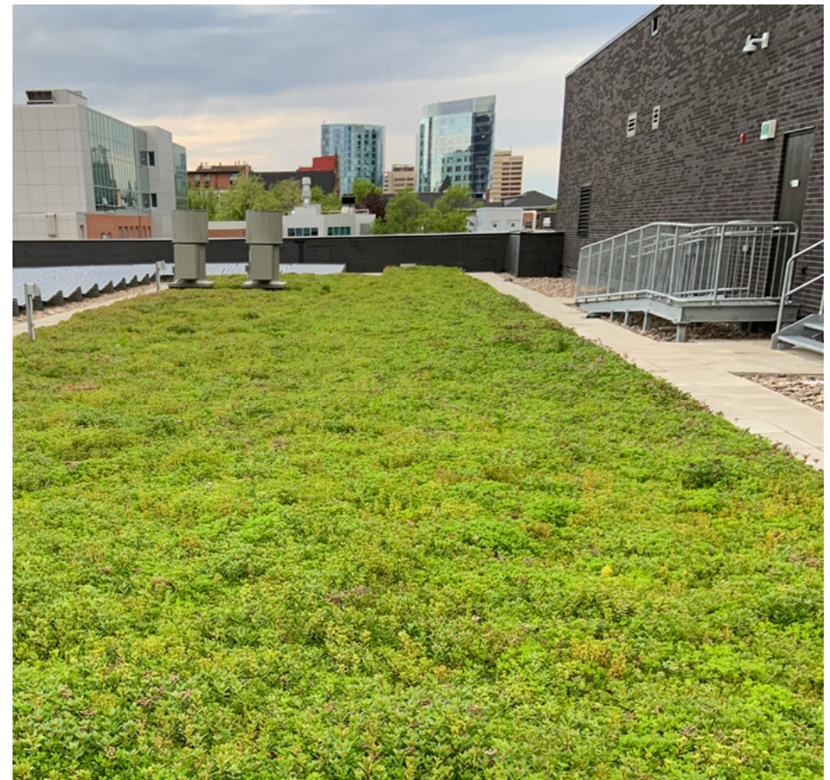
Photo 12. Green Roof on the Richard Murray Design Building.
