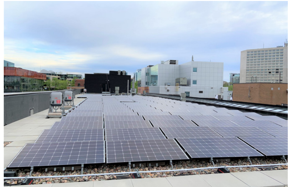
Photo 10. Solar PV panels on the Emera IDEA building.
