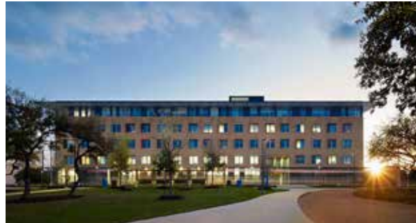
North Paseo Building
