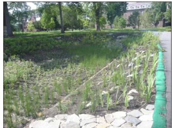
Figure 5 - Bio retention area near the Bridge Building at the former site of Mudd Laboratory
