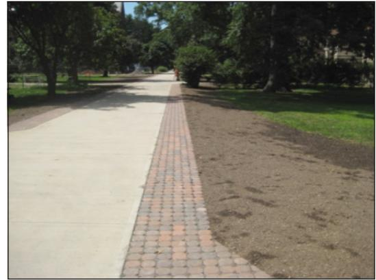
Figure 6 - Permeable concrete pavers on the residential quad
