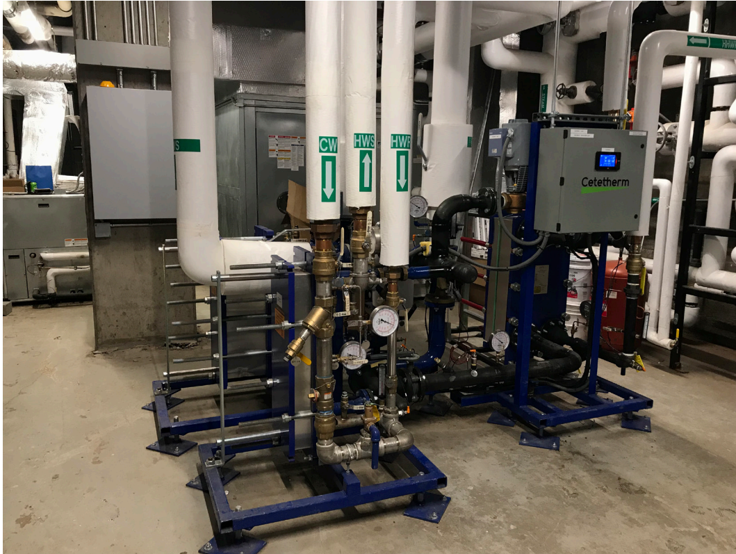
Figure 2. Typical district heating interconnection
