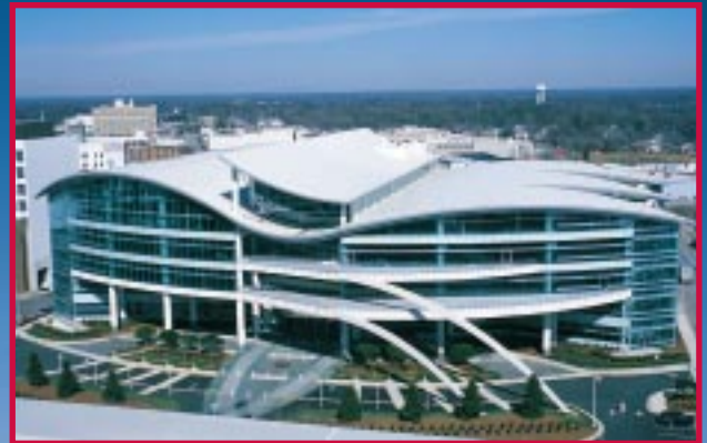
Showplace, High Point, North Carolina
