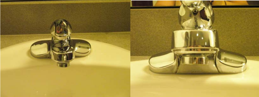
Delta faucet with 0.5 gpm vandal resistant outlet aerator attachment
