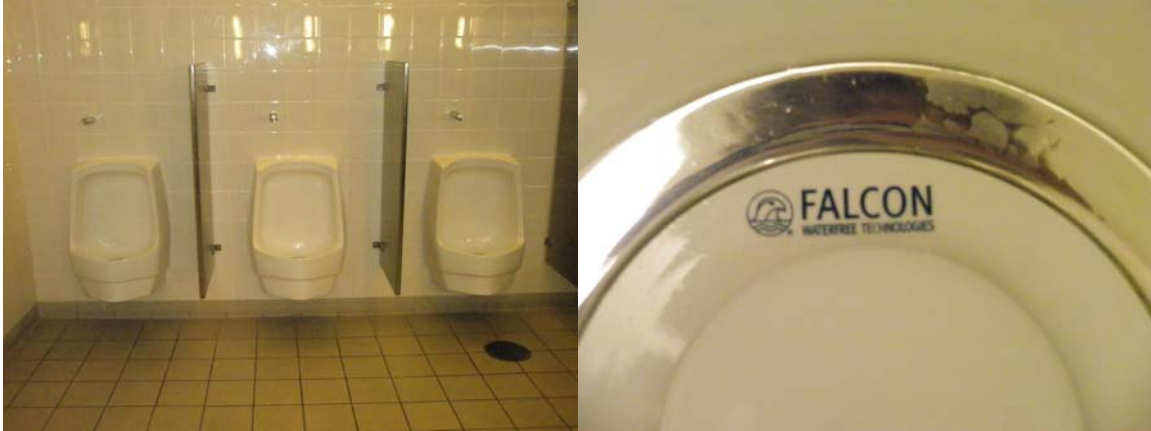
Falcon Technologies Water-free Urinals
