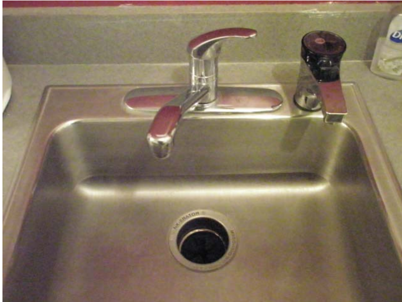
Symmetrix Single Hand Kitchen Faucet- 2.2 gpm flow rate Located in break rooms/kitchens on each floor of E2
