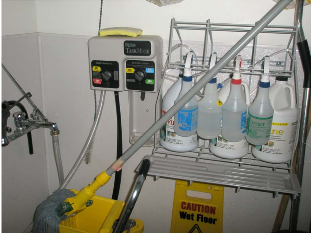
HYDRO CHEMICAL DILUTION SYSTEM
