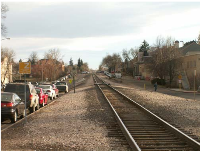
Railroad in ballast divides Mason Street.
