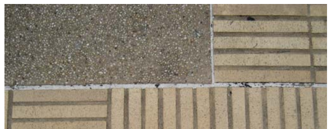
Heavily exposed aggregate concrete and brick pavers
