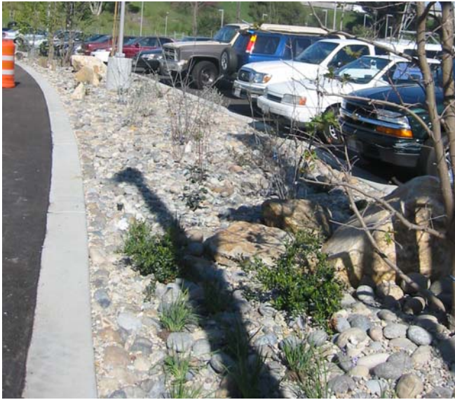
Bioswales in parking lots collect stormwater runoff allowing it some to soak into the ground, slowing flood conditions and adding character to the landscape.
