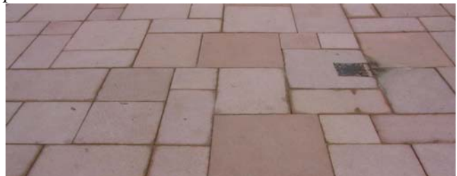
Precast concrete pavers in an ashlar pattern
