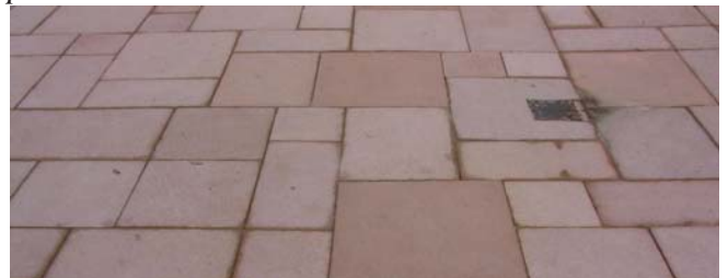
Pre-cast concrete pavers in an ashler pattern
