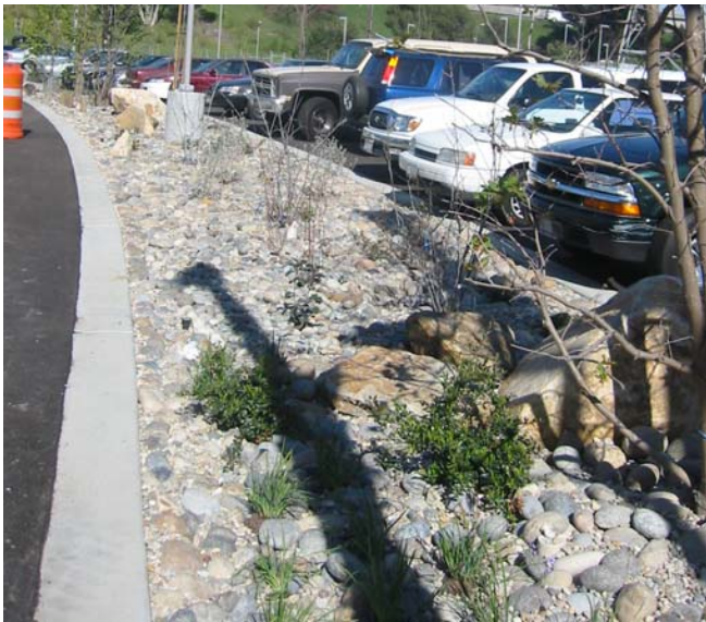
Bioswales in parking lots collect stormwater runoff allowing it some to soak into the ground, slowing flood conditions and adding character to the landscape.
