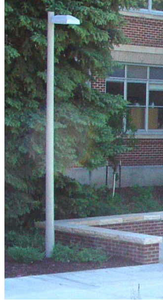
New light poles and fixtures used on the Main Campus should be used at the South Campus.
