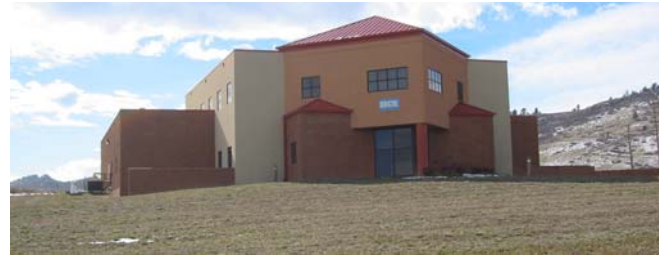
Site improvements are minimal at the Engineering Research Center.
