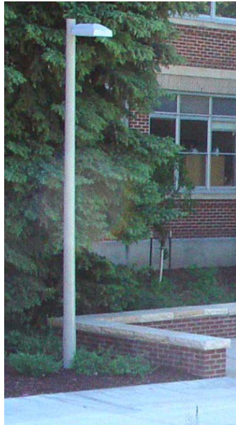
New poles and fixtures will replace the older lights.
