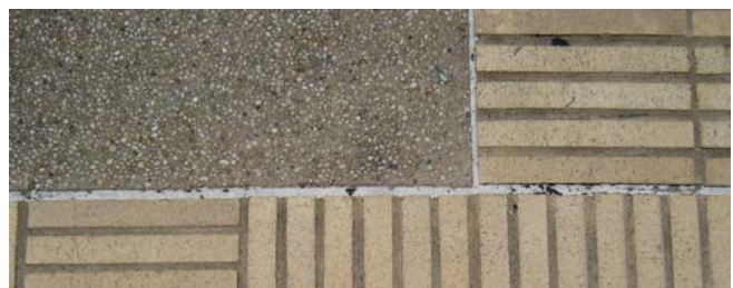
Heavily exposed aggregate concrete and brick pavers
