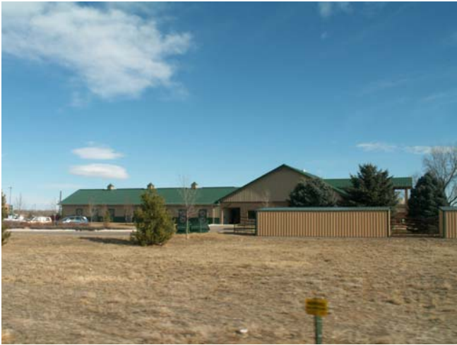
Large lawn areas surround the facilities at the South Campus
