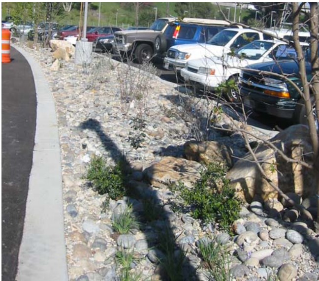
Bioswales in parking lots collect stormwater runoff allowing it some to soak into the ground, slowing flood conditions and adding character to the landscape.
