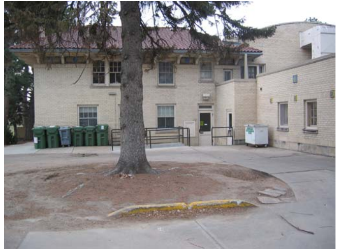
New understory planting would assist in screening the building services on the north side of Ammons Hall.
