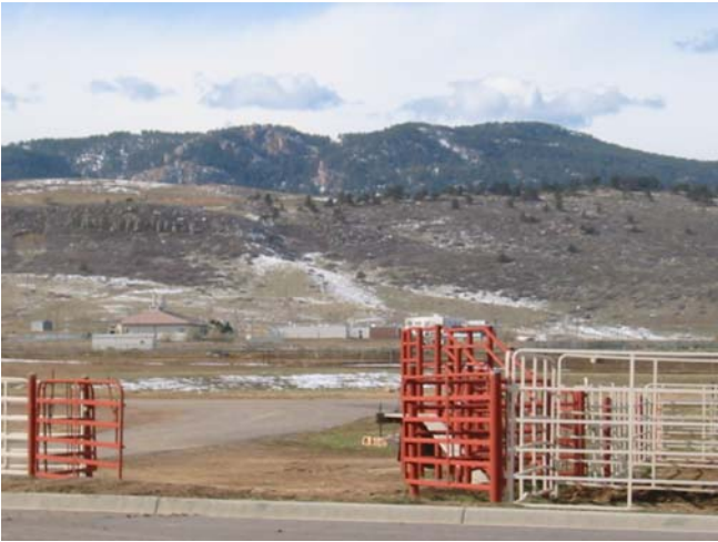
Pipe rail fence and gate structure enclose animal area.
