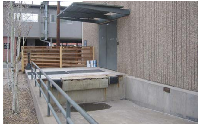
Trash and equipment is behind the horizontal screen.
