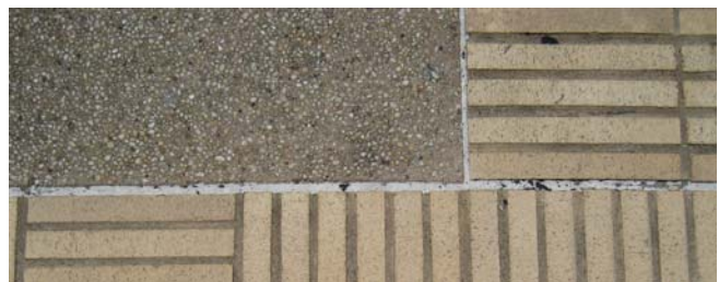
Heavily exposed aggregate concrete and brick pavers
