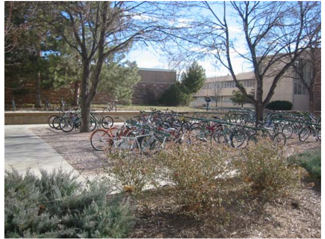
Bicycle parking along the Academic Spine is appropriately consolidated near building entrances, shaded and screened from view.
