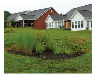
Figure 8: bioretention to capture sheet flow from neighborhood in Knoxville TN (Source: The SMART Center).
