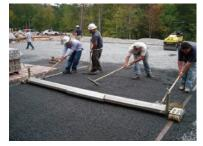
**Figure 24:** A 2 in. thick bedding course of aggregate is being screed smooth prior to placing the concrete pavers (Source: NCSU-BAE).
