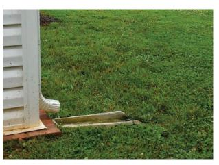
Figure 1: Roof downspout is directed to an infiltration area (Source: The SMART Center).
