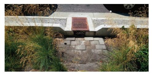
Figure 5.13: Paver inlet area of a bioretention cell that protects the media, dissipates inflow energy, and helps settle large solids for ease of maintenance.
