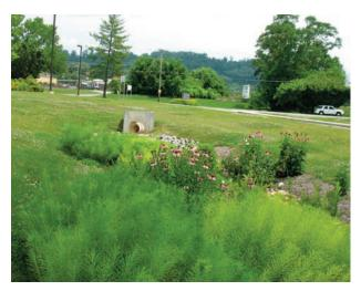
Figure 1: Bioretention capture water from parking lot in Powell, TN (Source: The SMART Center).
