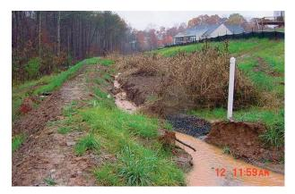
Bioretention swale, installed too early during active construction, has become clogged with sediment.
