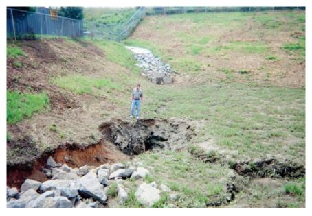
Figure: 7.1 Sinkhole Collapse in SCM.
