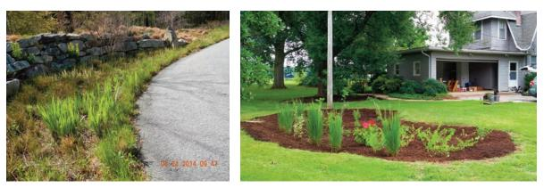
Figure 3.11: Photographs of lot scale runoff reduction measures. Left: a roadside vegetated verge (ie. no curb or gutter) that accepts roadway runoff, uses engineered soils to infiltrate runoff, and conveys excess runoff to a small treatment wetland. Right: a residential rain garden captures and infiltrates runoff from half of the house rooftop and driveway.
