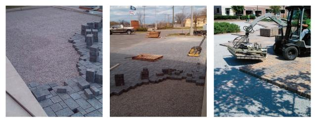
Figure 25: Alternative way of installing the permeable pavement (Source: R.K.).
