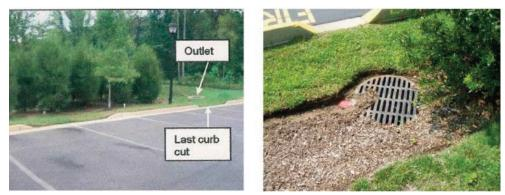
Figure 15: Short circuiting in bioretention (Source: VADCR).
