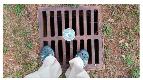
Figure 3.1: Stormwater management approach of storm drain stenciling, which identifies drains that discharge to local streams and states a no dumping regulation.
