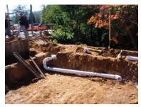
**Figure 21:** Installation of upturned underdrain and observation well (NC 2012, p:27).
