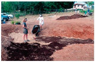
Figure 5.2: Soil amended with compost (Source: USDA NRCS).
