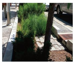
Figure 2: Street side planter boxes. runoff enters the planter boxes through curb cuts (Source: The SMART Center).
