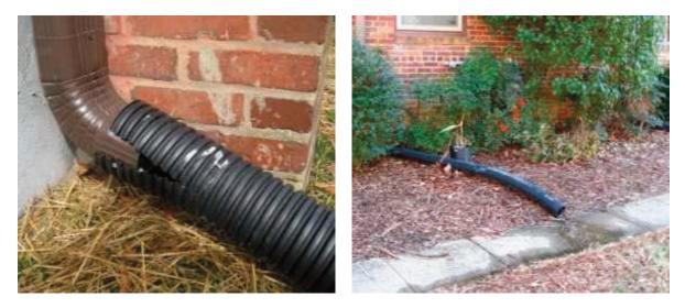
Figure 4: Poorly designed and installed downspout disconnections (Source: Carmen, NCSU).
