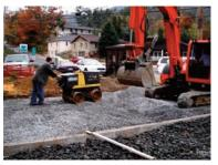
**Figure 23:** Compacting the open-graded aggregate base (Source: NCSU-BAE).
