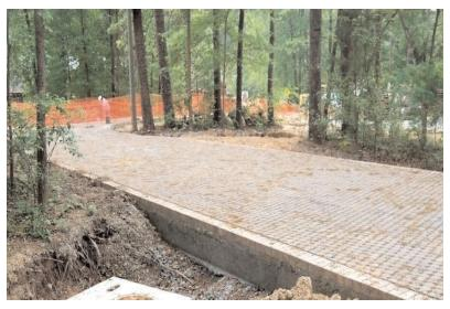
Figure 11: Edge restraint (Source: NCDENR).
