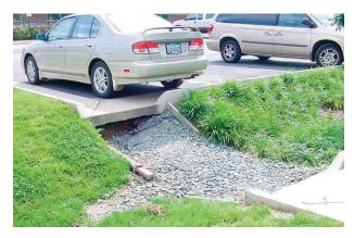
Curb inlets to bioretention swale have eroded because of improper sizing of stone.
