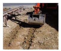
**Figure 18:** *Ripping the soil subgrade increases its infiltration rate (Source: Tyner).*
