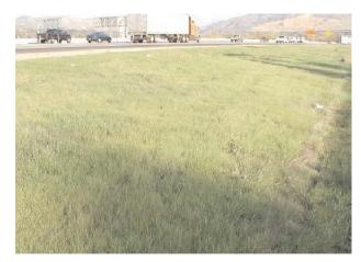
Figure 1: Filter strip along highway (Source: Virginia).
