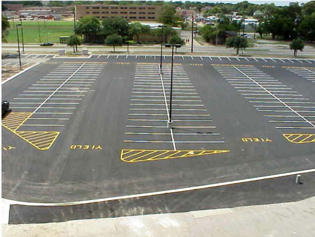
FIGURE 1.1 OVERVIEW OF PARKING LOT AND LIGHTING
