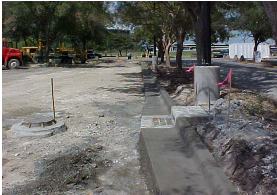
FIGURE 9.8.2 MONOLITHIC CURB, INLET AND CATCH BASIN
