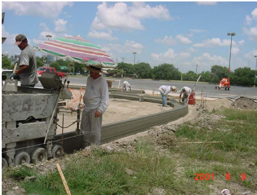
FIGURE 9.2.8 MONOLITHIC CURB ALONG PERIMETER OF PARKING LOT
