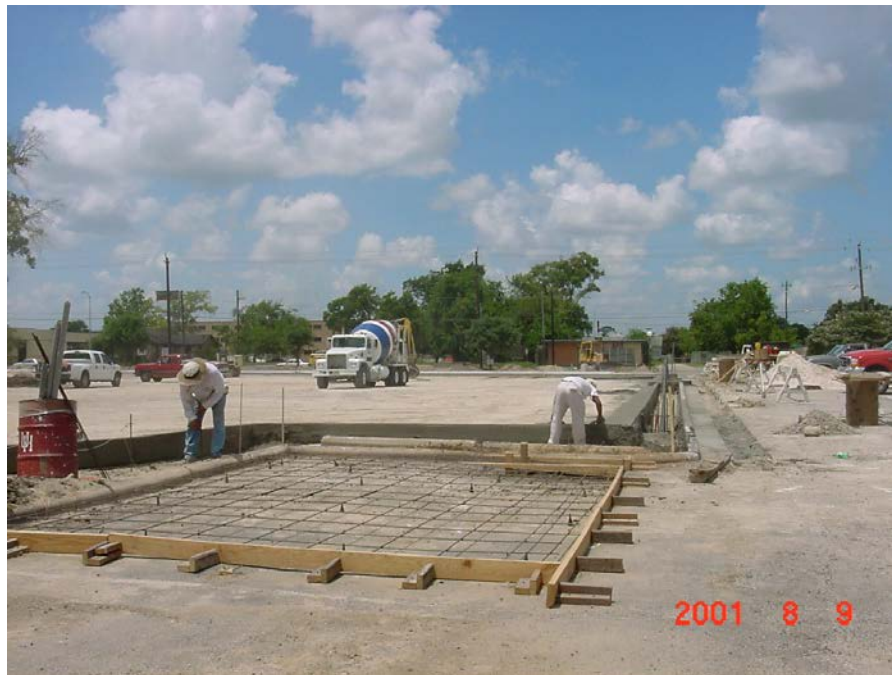
FIGURE 9.6.1 FRAMING AND REINFORCING FOR CONCRETE PAD
