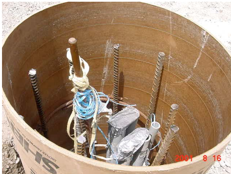
FIGURE 9.9.4 REBAR, ELECTRICAL CONDUIT
