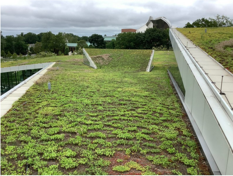
Overall view of the green roof (facing north).
