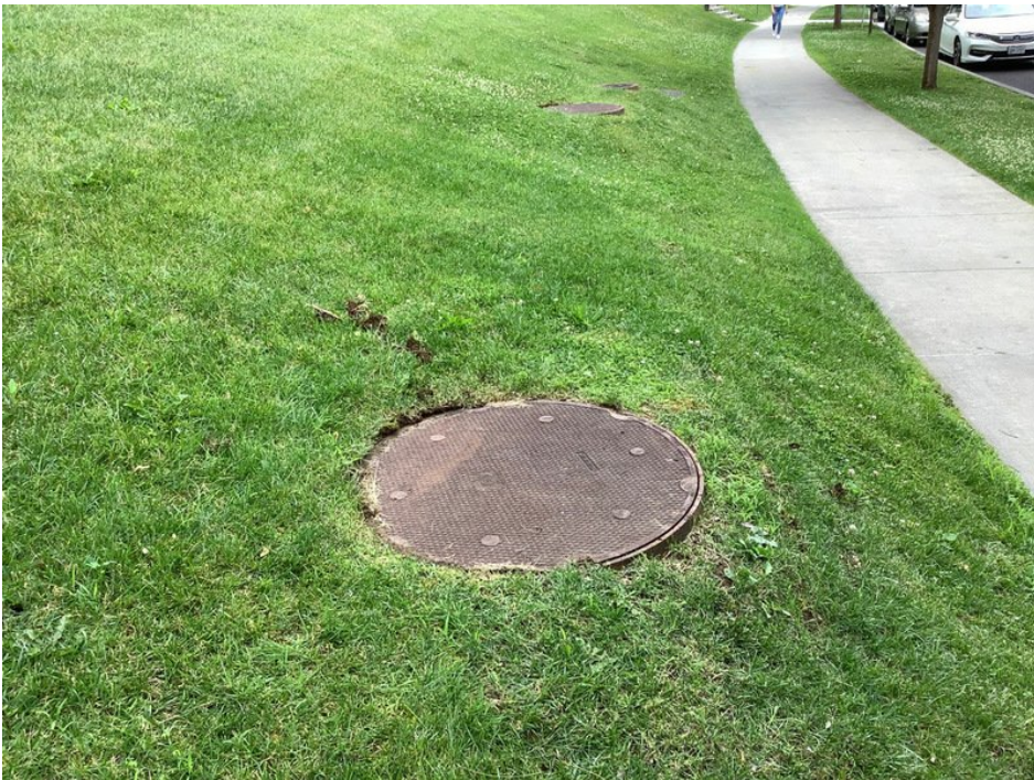
Overall view of the location of the sand filter (facing west).
