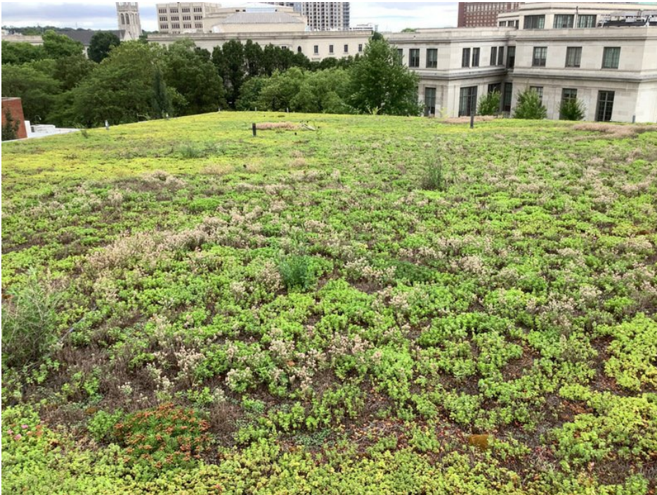
Overall view of the south section of the green roof (facing
