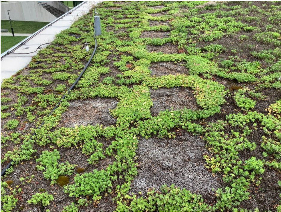
View of dead vegetation on the southwest side of the green roof due to past maintenance activity.
