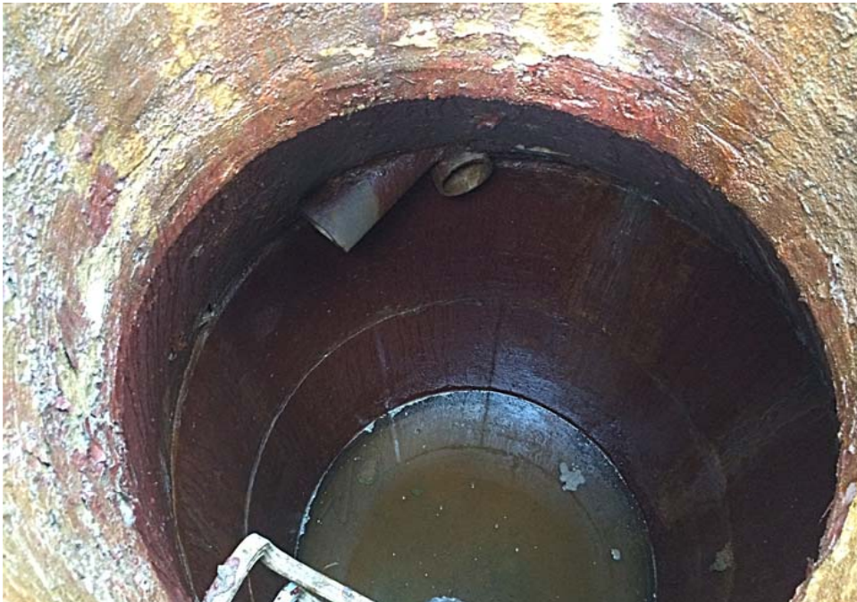
West Tank Before Cleaning
