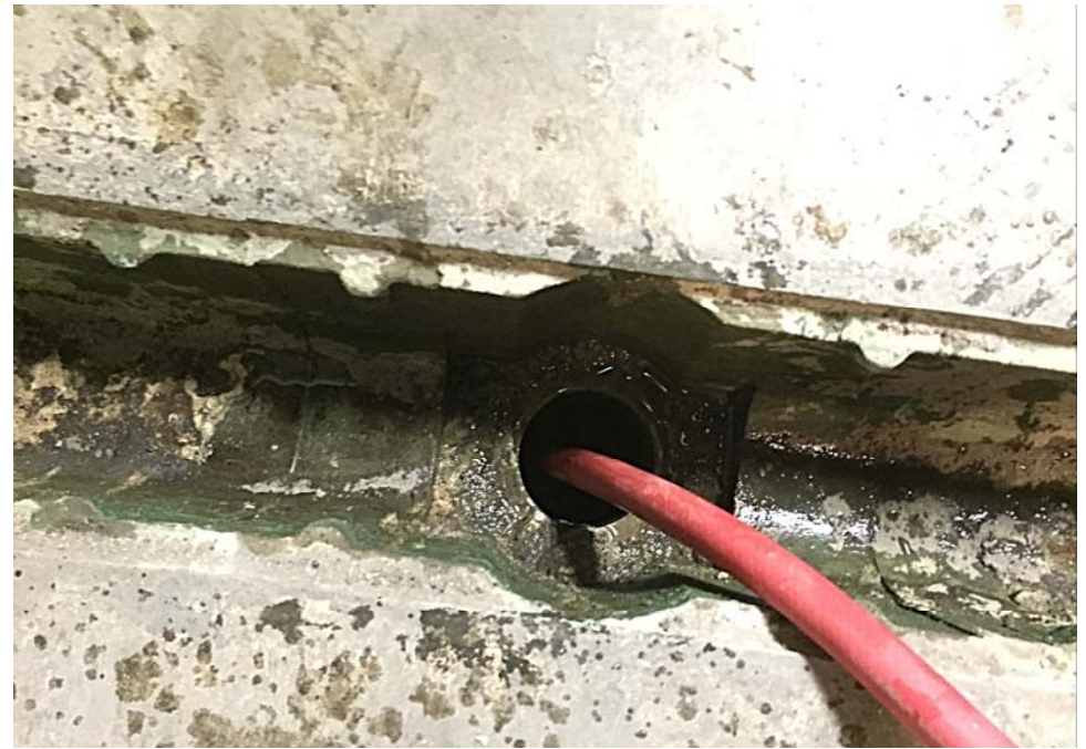
Drain Jetting Process
