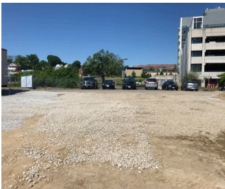
Install a construction access pad
