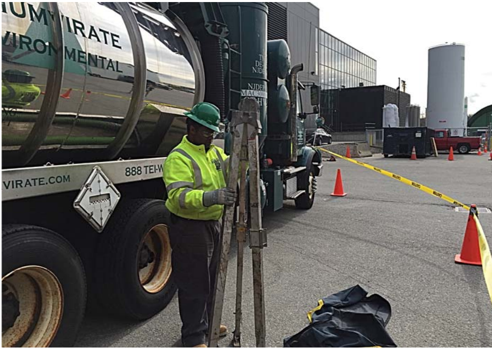
Confined Space Entry Set-Up
