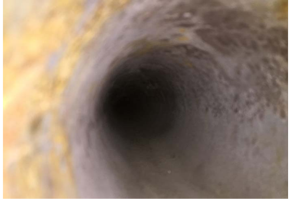
Tank Vent Pipe Inspection
