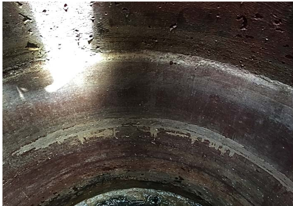
East Tank Walls Following Liquid Removal
