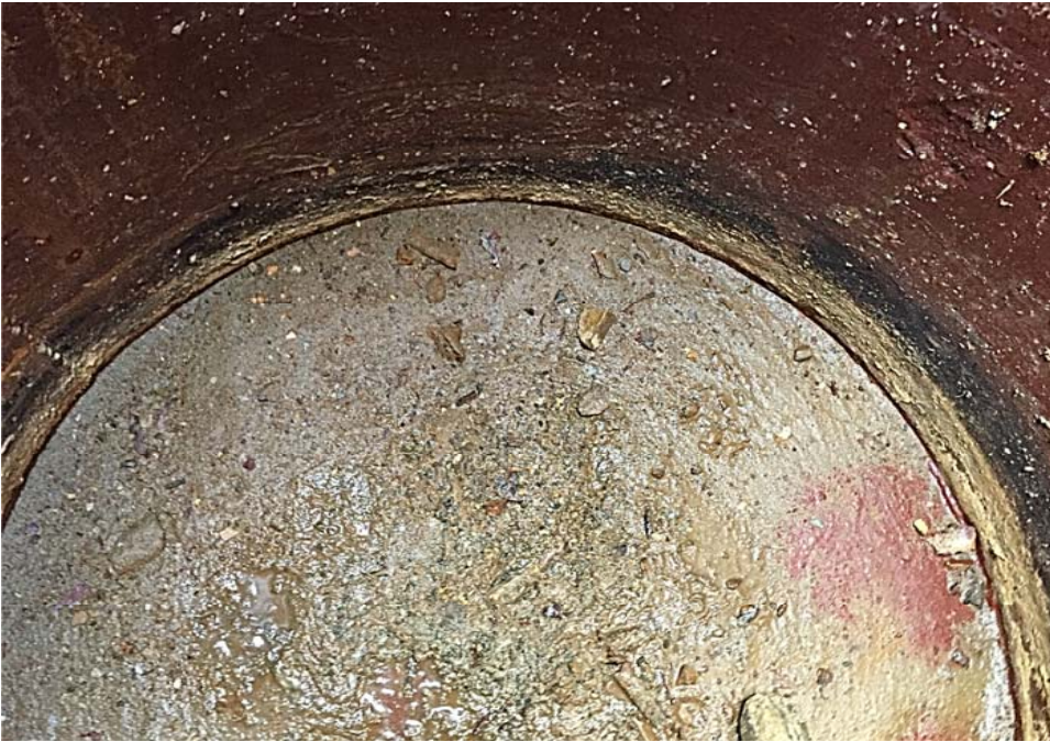
West Tank Bottom Following Liquid Removal. Sediment Remains
