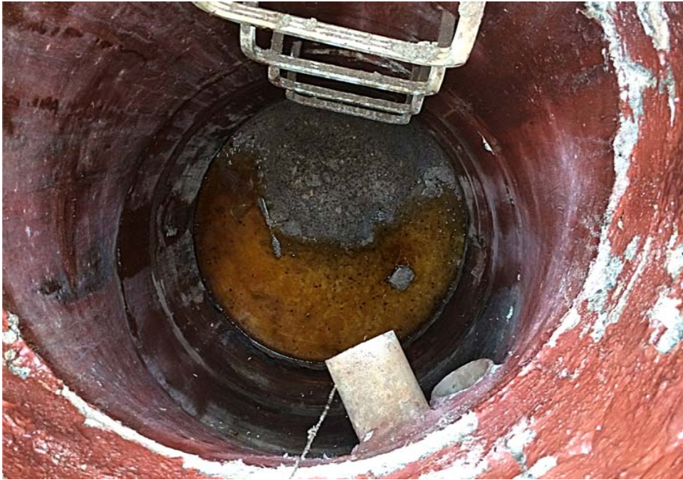
East Tank Before Cleaning
