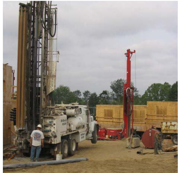
Drilling Geo-Thermal Wells, Northwoods Village Apartments
