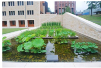
Figure 3.6-1: LEED Platinum Kroon Hall at Yale University. Within this rainwater harvesting system, aquatic plants like iris, cattails, arrowweeds, and lotuses cleanse runoff in a stormwater basin through phytoremediation (Photo credit: Landscape Architecture Foundation).
