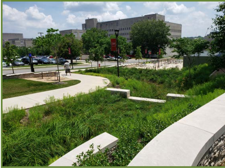
In this example, Indiana University has incorporated a highly functional bioswale as the main focal point of one building's foundation landscape.
