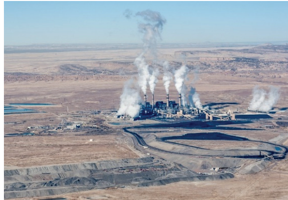
The San Juan Generating Station near Farmington, N.M. Credit: Sierra Club, courtesy of Ecoflight
