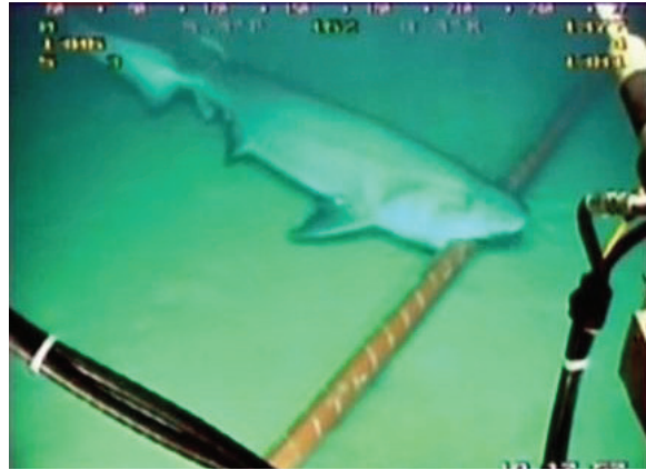
Video footage of a shark biting an undersea cable. While sharks and other marine life can damage fiberoptic cables, incidents are rare. Credit: Michael Graham Richard, TreeHugger
