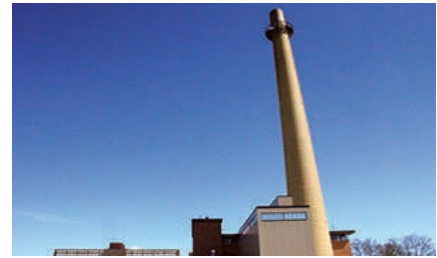
UW- Eau Claire's Steam Plant - Spectator
