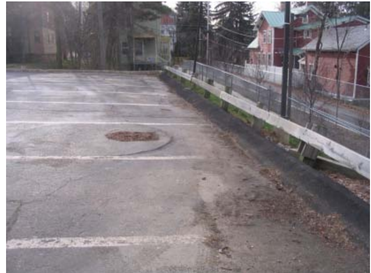
CB grate filled in with leaves
