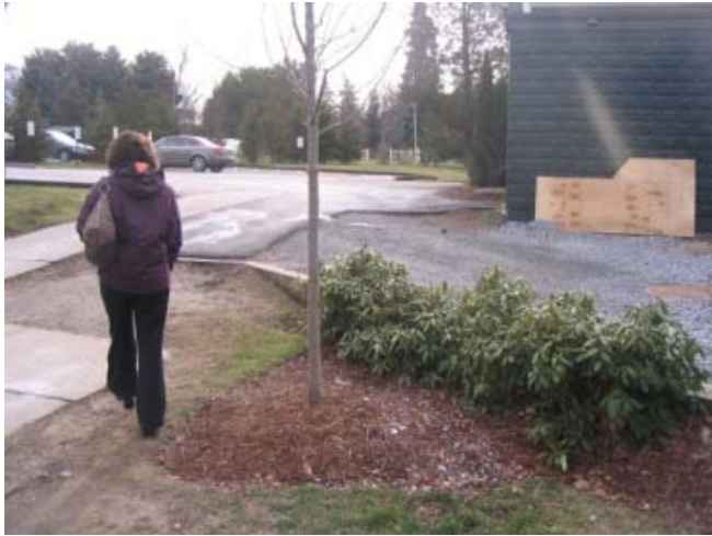
Area near Carriage House Poorly graded area
