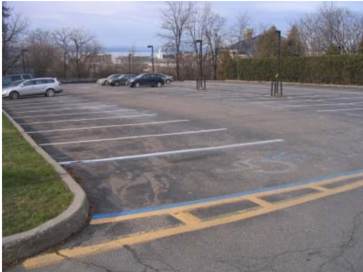
McDonald Hall/Whiting Hall parking lot: Large impervious area w/ no CB's or disconnection of runoff
