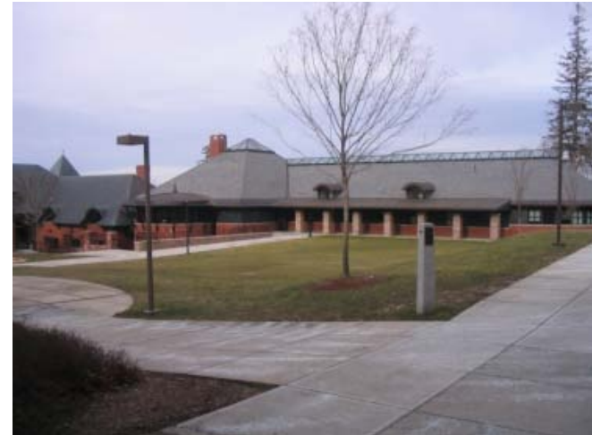
S.D. Ireland Center, from campus green
