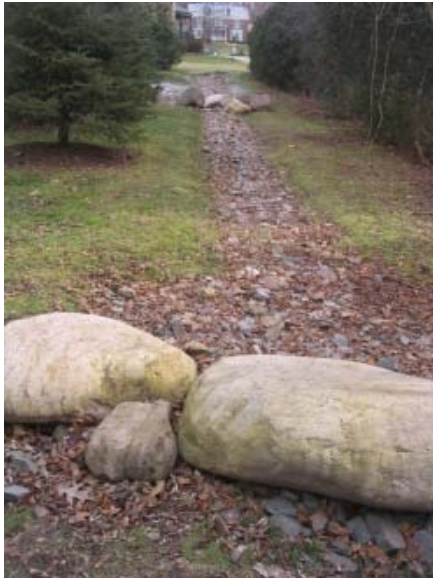
Stone drainage swale w/ boulder check dams
