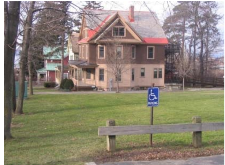
Goodhue-Coolidge House (wet basement at times)
