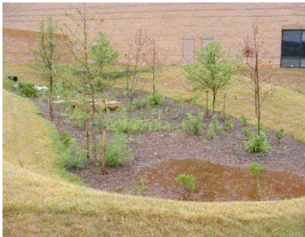
STORMWATER BIORETENTION POND
