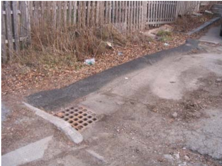
Catch basin at end of Harrington Terrace
