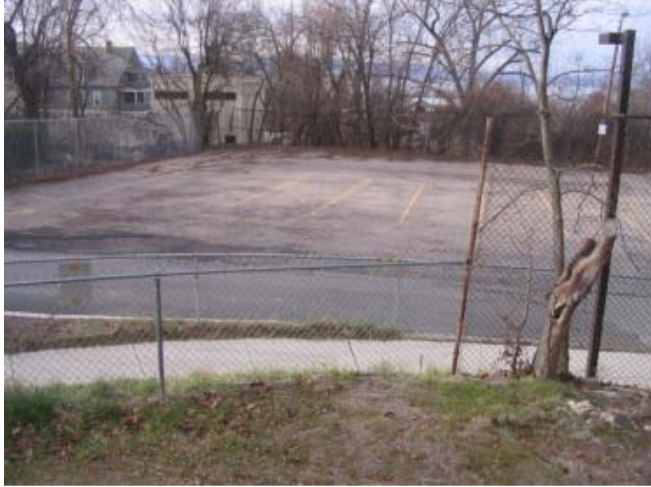
Adjacent Edmunds School parking lot: Large impervious area w/ no CB's or disconnection of runoff
