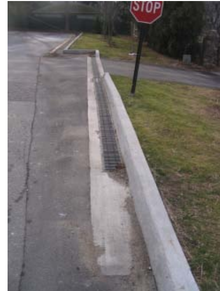
Trench drain collecting runoff to discharge into stone drainage swale
