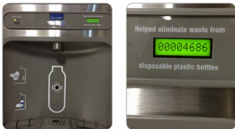
Figures 47 & 48: UNO has added several water bottle refill stations across campus. Students and employees enjoy using the stations because they help eliminate waste in the form of disposable plastic water bottles. In fact, each station displays a running count of how many disposable plastic water bottles it has displaced.
