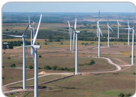
Figure 39: OPPD gets some of its energy from the Flat Water Wind Farm in Richardson County. As OPPD continues to increase its renewable energy profile in the coming years, UNO will become closer to its carbon neutrality goal (photo credit: OPPD)
