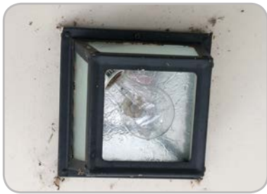
Figure 35: UNO should replace all incandescent bulbs, like this one at University Village, with CFLs or LEDs. The payback period for a CFL is typically less than 12 months while the payback period for a LED can range from 12 - 36 months.
