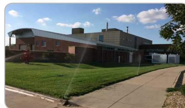
Figures 44 & 45: Opportunities exist for UNO to ensure it is only watering turf grass during appropriate times. For example, these photos were taken during the middle of the afternoon on hot summer days; watering during these conditions is not ideal.
