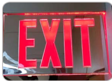
Figure 36: UNO should expect noticeable energy savings by replacing its older exit signs with newer ones that utilize LED technology.
