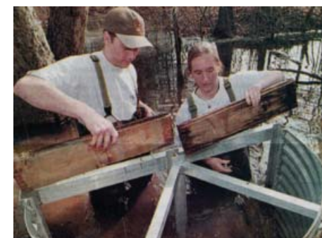
Students stem the flow of water with boards for the waterfowl impoundment.
