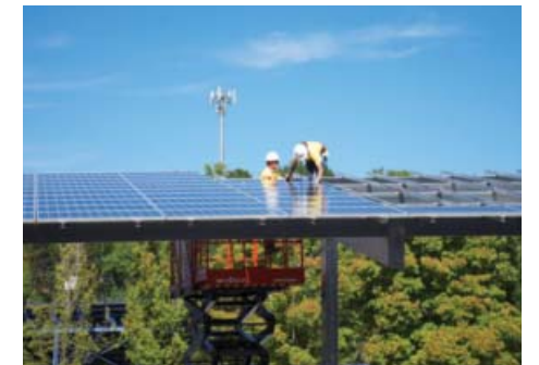
Workers install solar panels over the athletic field parking lot.
