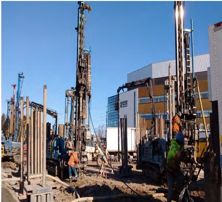
Picture 2. Geothermal System Construction
