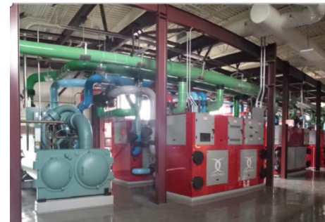
York Variable speed Magnetic Bearing Chiller (green) and Chillit Heat Pump Chillers (red).
