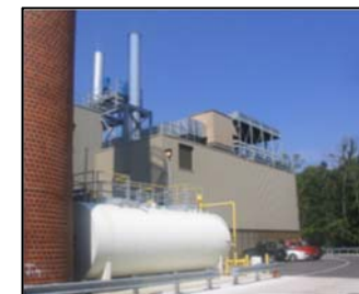
Steam Plant building addition that houses the Peaking Engines.
