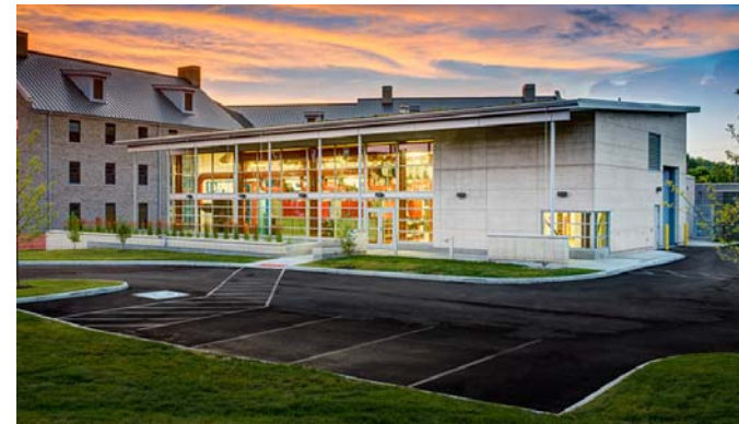
The Western Geothermal Plant.
