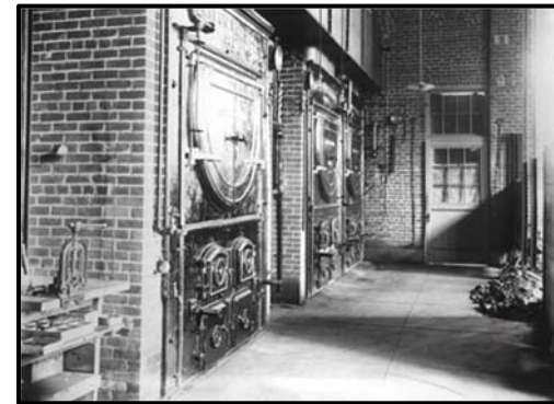
Furnace Room, Central Heating Plant 1907.
