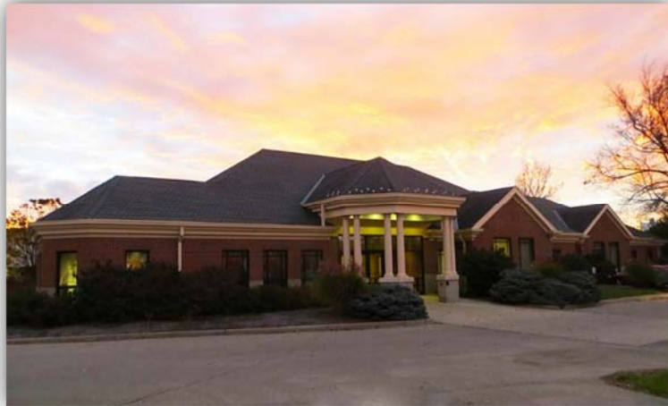
All Utility Systems are managed by the engineering group and maintenance staff, located in the Cole Service Building.
