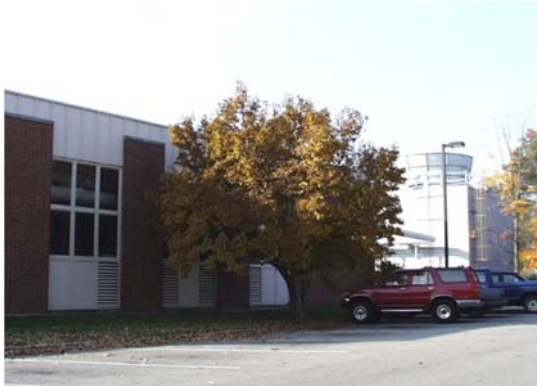
The South Chiller Plant.
