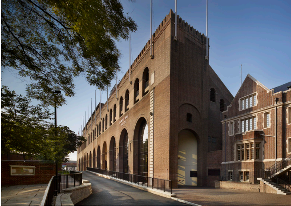
Porous pavements at Weiss Pavilion
