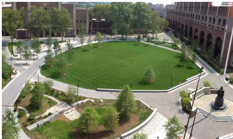
Porous pavements at Weiss Pavilion and Shoemaker Green
