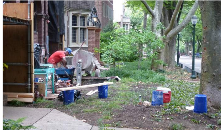
Figure 3.4 - Recently planted beds used for staging.
