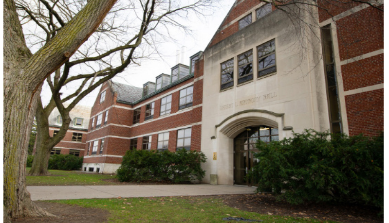
A photo of Anthony Hall, which was outfitted with Aircuity installations along with six other campus buildings.
