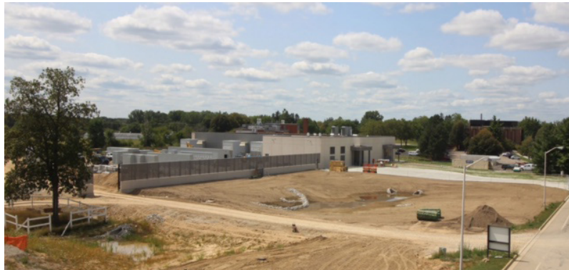
Construction progress as of August 25, 2017 on the MSU central data center.
