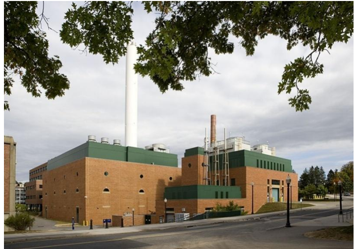
Figure 3.1. The UConn cogeneration facility. The facility went online in mid-2006 and will serve as the primary energy source for the next 30-40 years.
