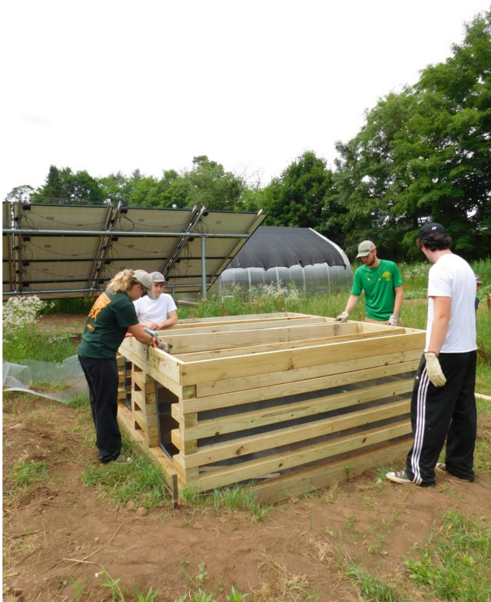
Students and volunteers constructing the crib portion of the composting privy. (Courtesy of Eliza Cochrane)
