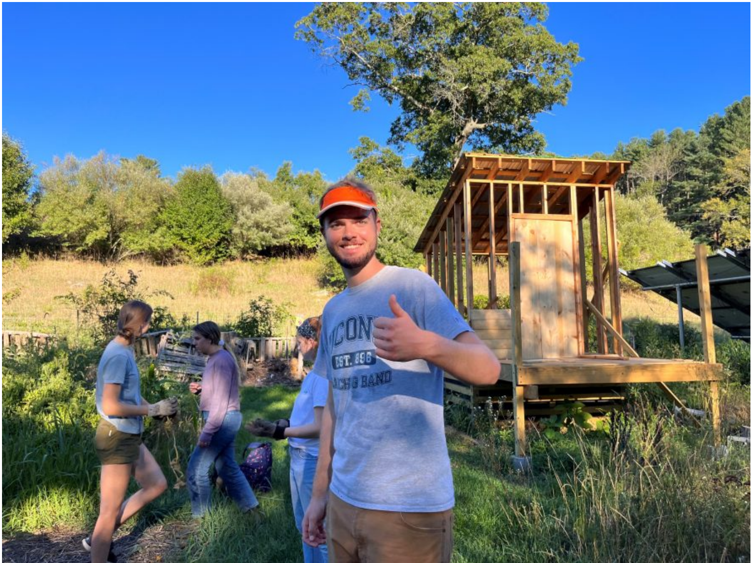
Students pose in front of the composting privy. Construction will be completed in the near future. (Courtesy of Rory Monaco)
