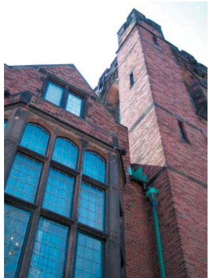
North elevation, downspout 1
