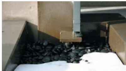
(Above) Downspout splash block and catch basin, Epler Hall Dormitory Plaza, Portland State University. (Below) Infiltration beds, Epler Hall Dormitory Plaza. Water runs in stone runnels between the downspout and beds. Unlike a typical rain garden, water passing through the beds is collected and used to flush toilets in the building.
