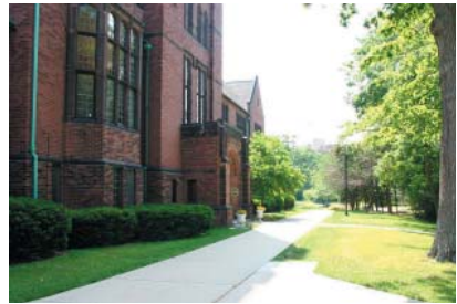
North elevation, downspouts 1 & 2
