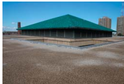
Roof opening to fountain area below
