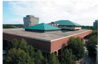
Looking northeast, from the roof of the business building.
