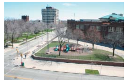
(Below) Existing condition- Sidewalk and retaining wall at the corner of Hartford and Maryland, looking east.
