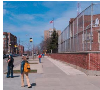
(Above) Existing condition- Maryland Avenue sidewalk and retaining wall, looking north.
