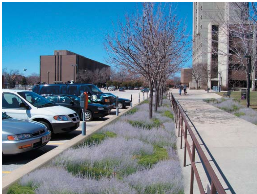
HYPOTHETICAL LINEAR RAIN GARDEN An existing grade change is used to capture sidewalk run-off
