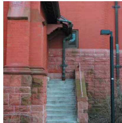
Merrill Hall, downspout 9.
