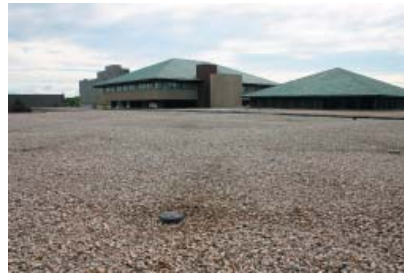
From the northwest corner, looking southeast.
