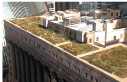
Chicago City Hall green roof. Conservation Design Forum, Landscape Architects.
