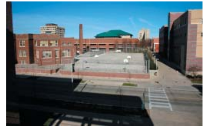
Existing asphalt playground and retaining wall. Looking east from the School of Architecture and Urban Planning.
