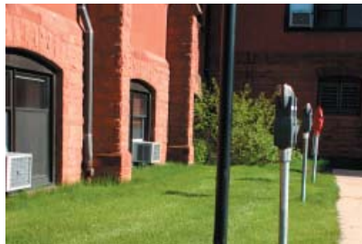
Merrill Hall, downspout 4.
