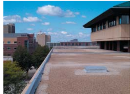
Southern roof area, looking west
