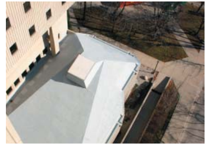
South lecture hall roof from above. Downspout 5 through 9.
