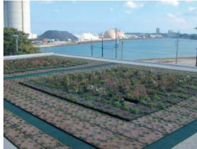
UWM Water Institute Green Roof
