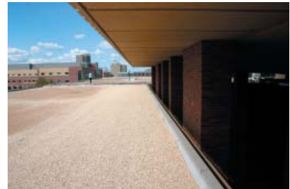
Overhang condition at central pavilion over library mall.
