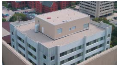
Roof, East Tower, viewed from the roof of the North Tower. Only the newly constructed East Tower suggests the potential for a green roof application.
