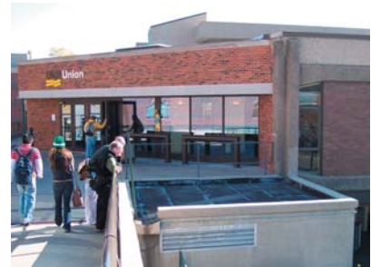
(Above) View of roof as is. (Below) View of roof with hypothetical green roof installation.
