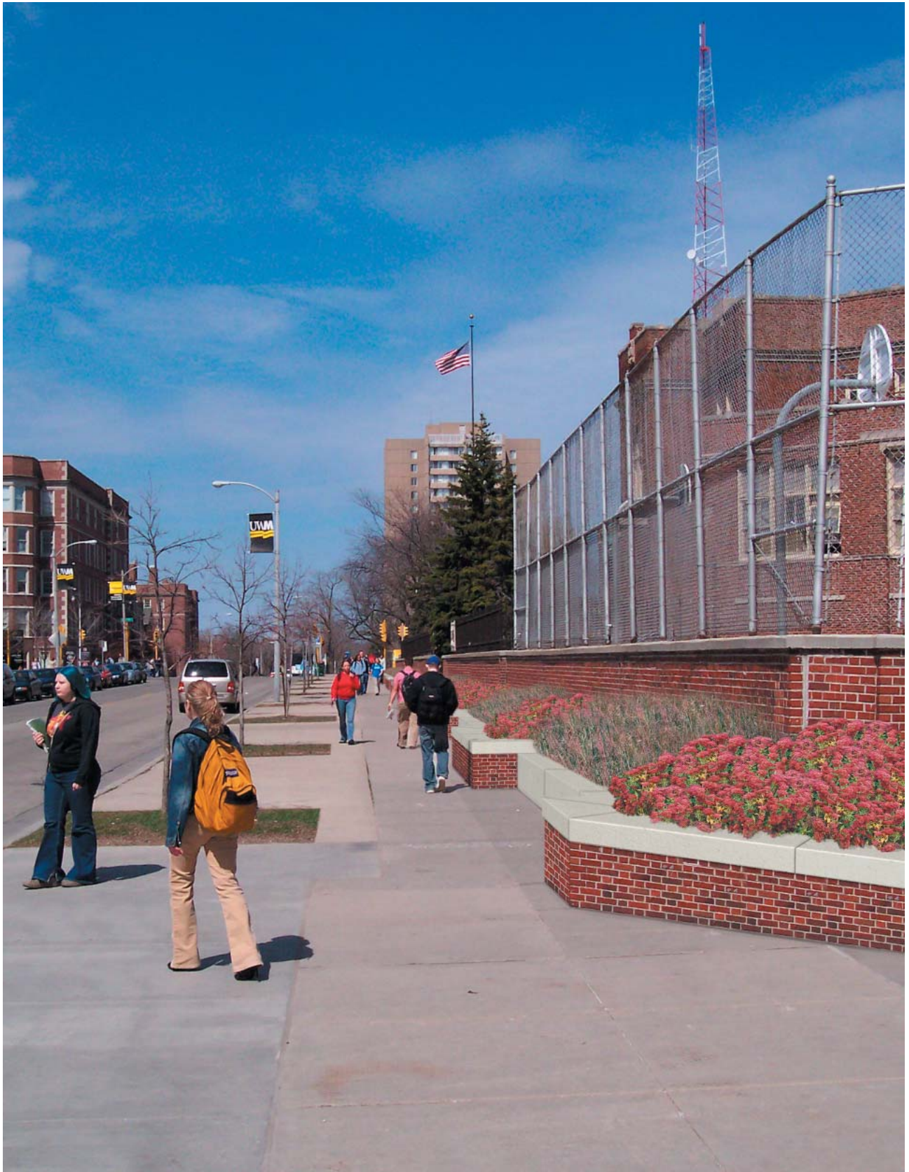
HYPOTHETICAL HARTFORD AVE. SCHOOL PLANTER BENCH A rain garden planter draining the Hartford Ave. School playground
