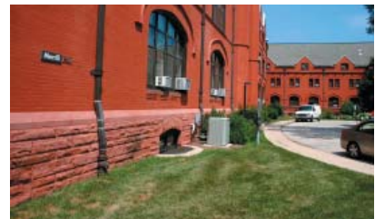
Merrill Hall, south facade, downspouts 14, 15 and 16.
