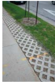
Grass Paver Blocks, Prospect Avenue, Milwaukee.
