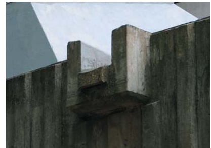
Expressed roof scupper.
