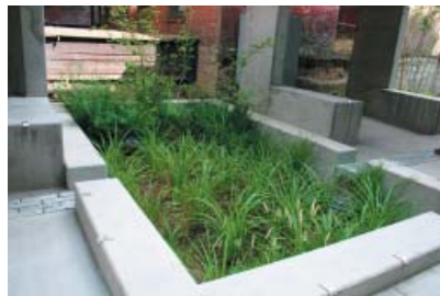
(Above) Downspout splash block and catch basin, Epler Hall Dormitory Plaza, Portland State University. (Below) Infiltration beds, Epler Hall Dormitory Plaza. Water runs in stone runnels between the downspout and beds. Unlike a typical rain garden, water passing through the beds is collected and used to flush toilets in the building.
