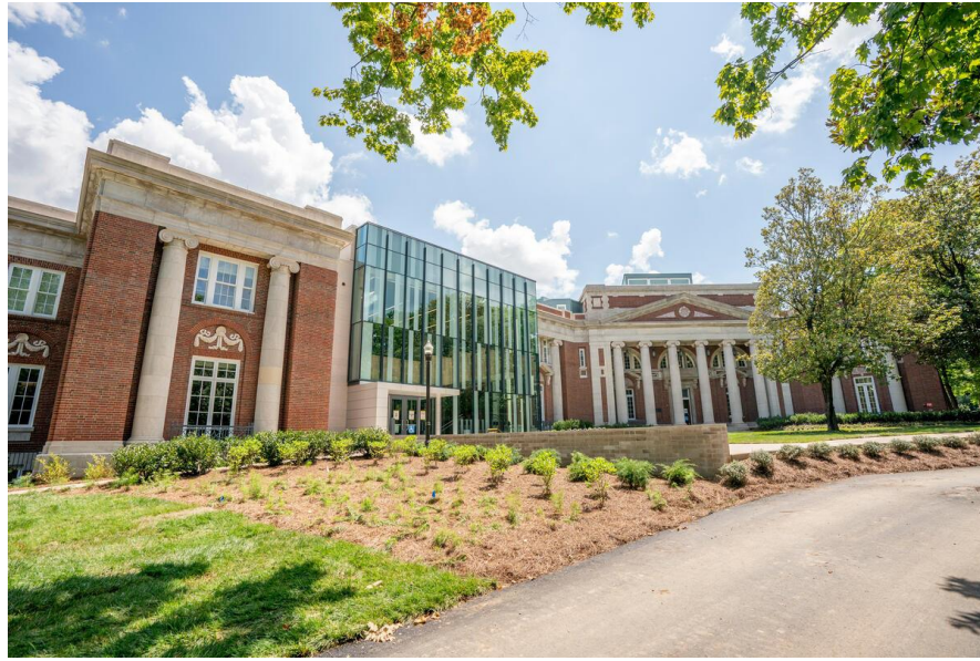
Figure 18 6 Magnolia building, Vanderbilt's first building designed with a Living Building Challenge Petal Certification
