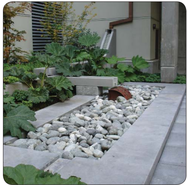
Fig. 4.21 Flow-Through Planter Box in Portland, OR (JJR)
