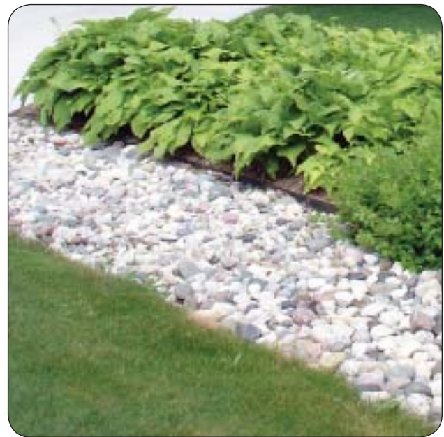
Fig. 4.17 Infiltration Trench Incorporated Into Landscape (JJR)
