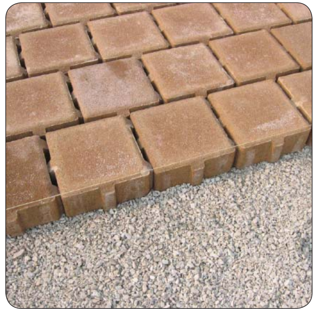
Fig. 4.10 Permeable Pavers Installed at Recreational Sports Field, August 2007 (JJR)
