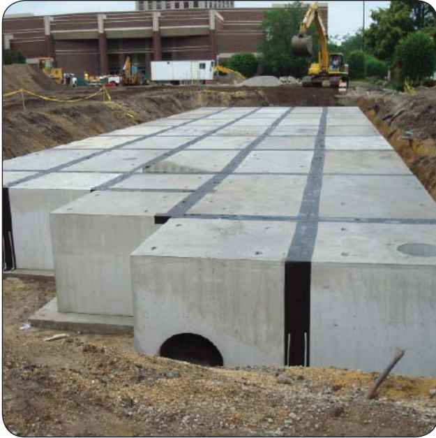
Fig. 3.3 StormTrap® - Lake Shore Campus, June 25, 2008 (JJR)
