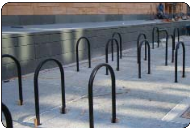
Fig. 4.13 Porous Concrete Bike Parking - Under Construction at University of Michigan (JJR)
