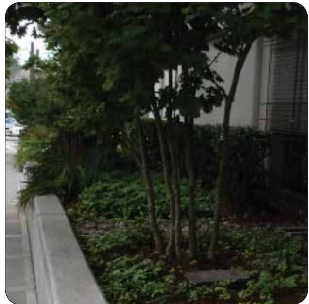
Fig. 4.22 Flow-Through Planter Box in Portland, OR (JJR)
