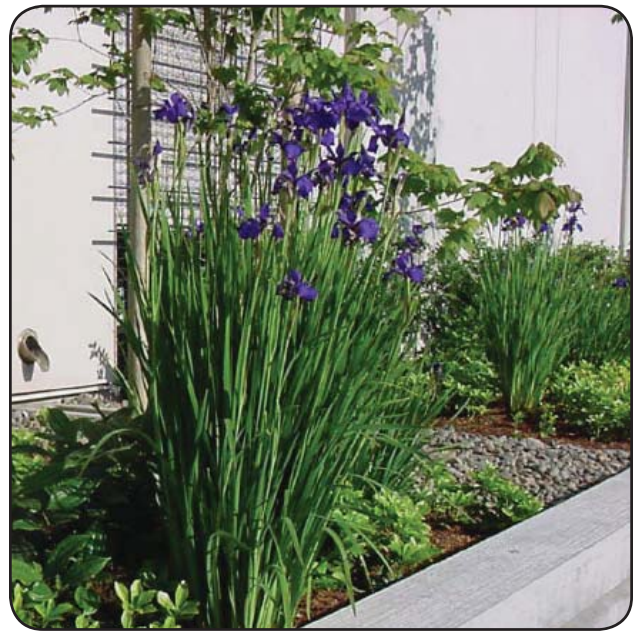
Fig. 4.25 Flow-Through Planter Box in Portland, OR (Portland Stormwater Management Manual, Revisions, September 1, 2004, www.portlandonline.com/bes)
