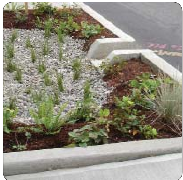
Fig. 4.18 At-Grade Infiltration Basin in Portland, OR (JJR)
