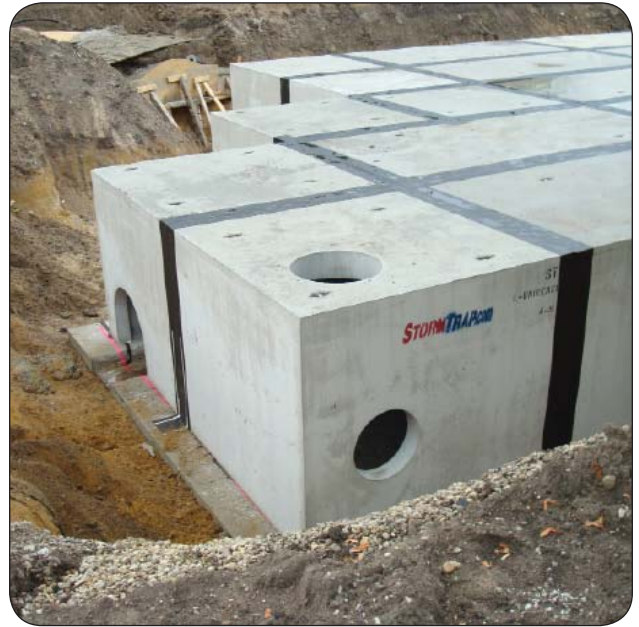
Fig. 3.4 StormTrap® - Lake Shore Campus, June 25, 2008 (JJR)
