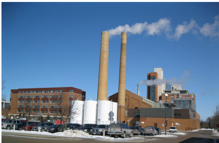
Figure 1: U of M Central Energy Plant
